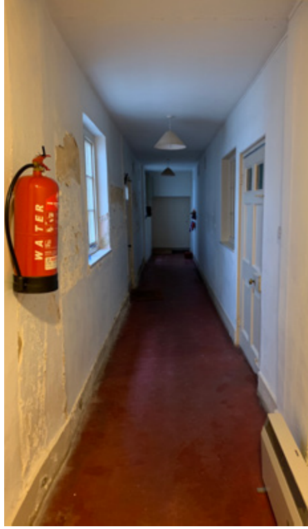
Red Passage in Salvin's rebuilt range. View facing west.
