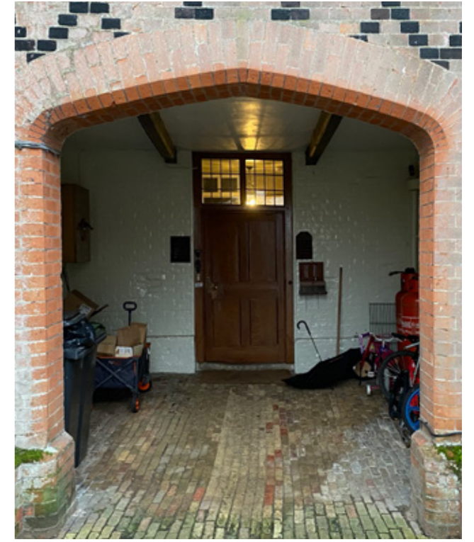
Proposed area for new boot room - view facing west
