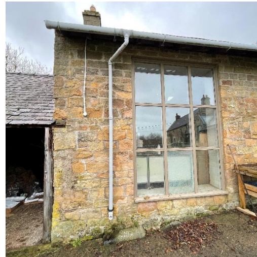
Figure 5 – Modern openings in West wing
