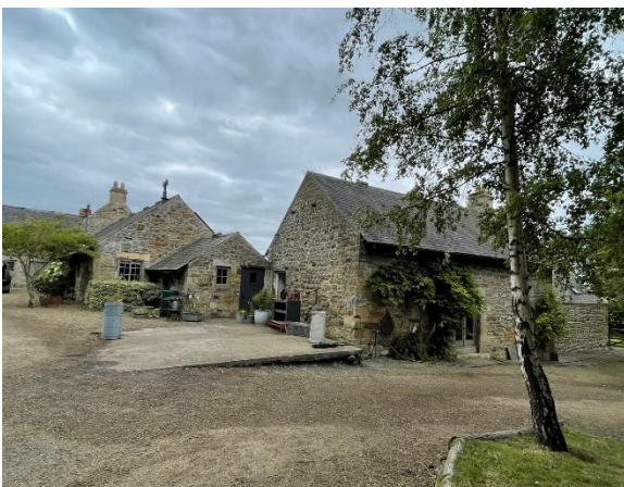
Figure 4 – West wing & former coal shed slab
