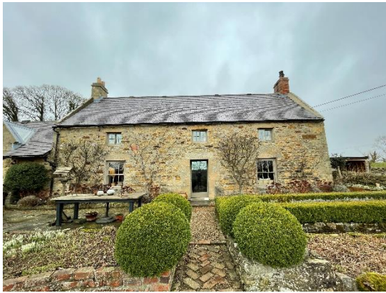
Figure 10 – North Farmhouse G II Listed
