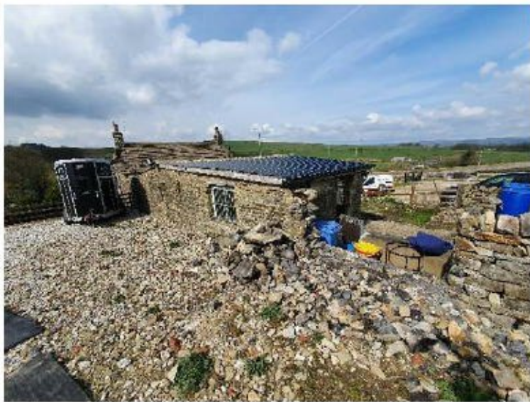
Existing stable block
