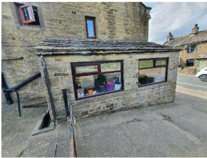
Existing lean-to extension
