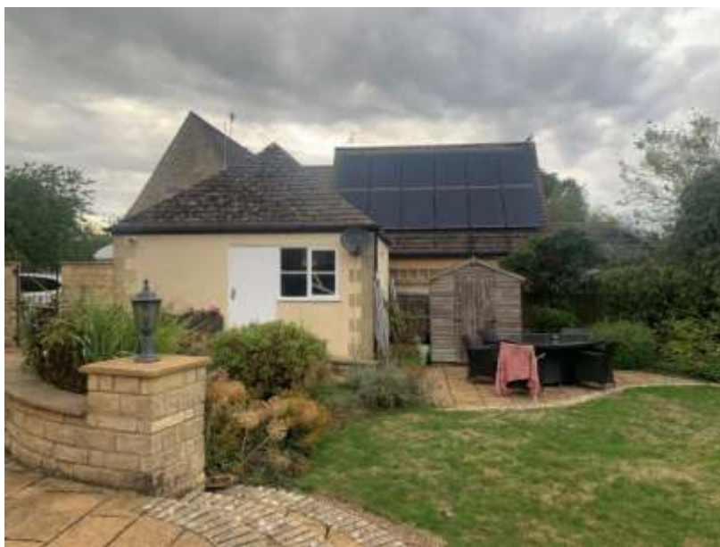
Figure 4 – Existing Garage Block
