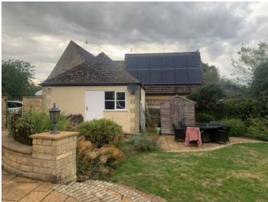
Figure 4 – Existing Garage Block
