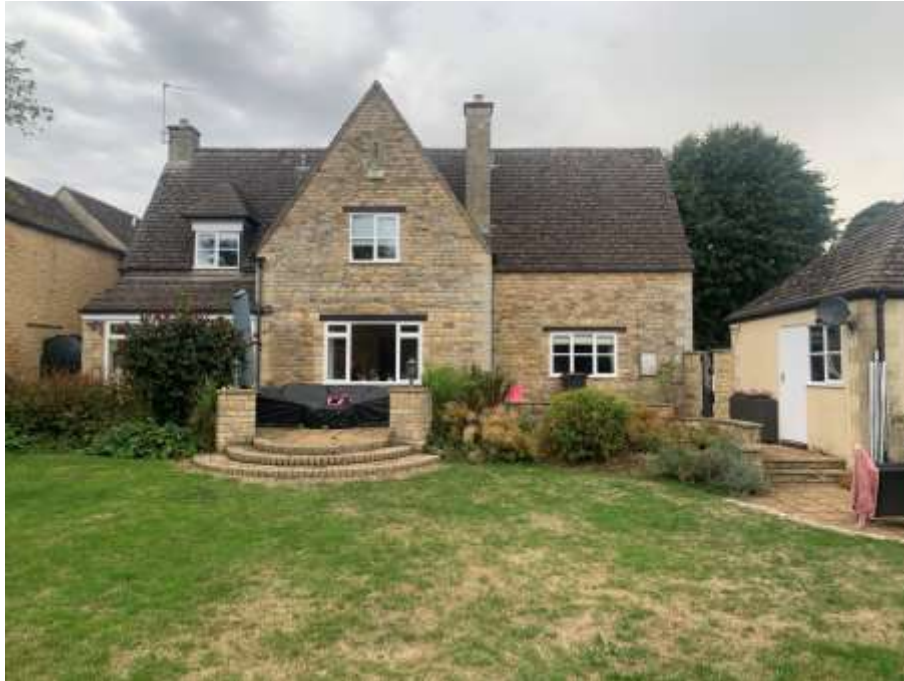
Figure 3 – Existing Rear Elevation
