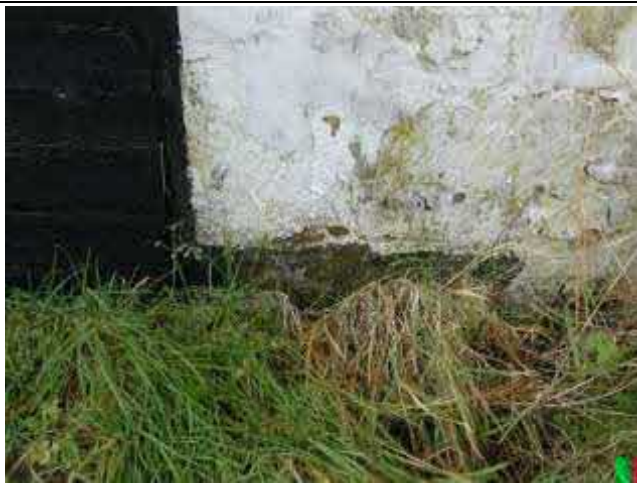
Join Between Cottage Extension and Garage
