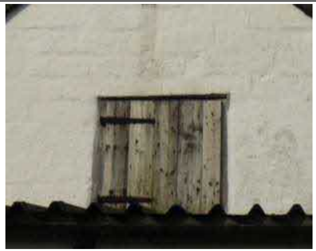
Timber Door at First Floor to East Elevation
