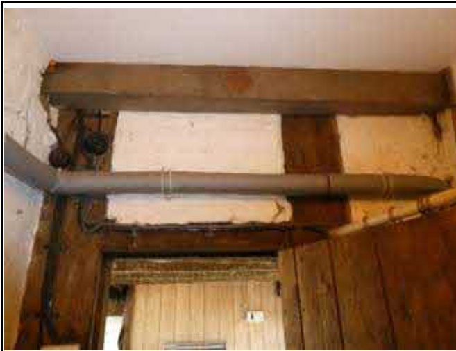
Metal Pipe on the West Wall
