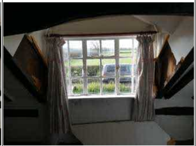
Window to the South Wall
