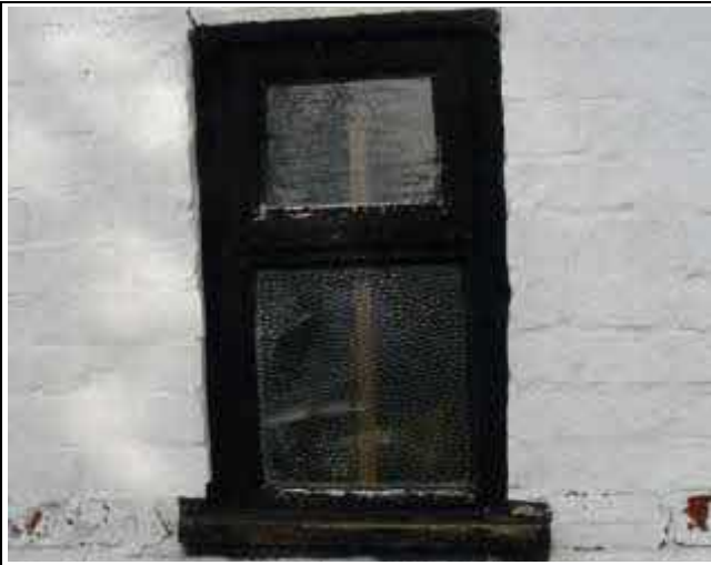
Small Window to East Elevation
