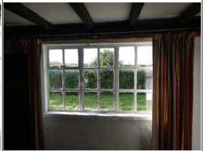
Timber Window to the Front
