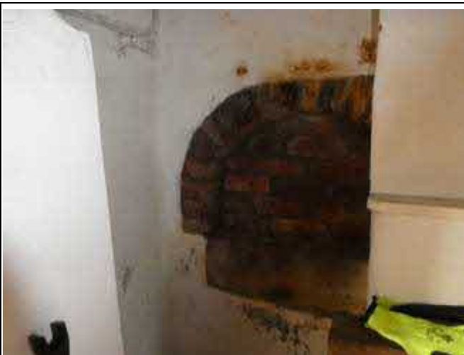
Sealed Brick Arch
