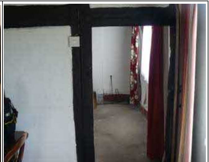
Door Frame to Kitchen
