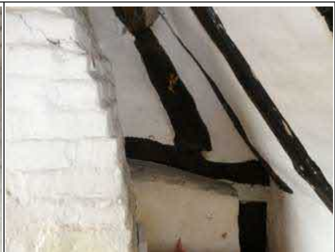
Exposed Tiebeam and Rafter on Either Side of the Chimney Breast
