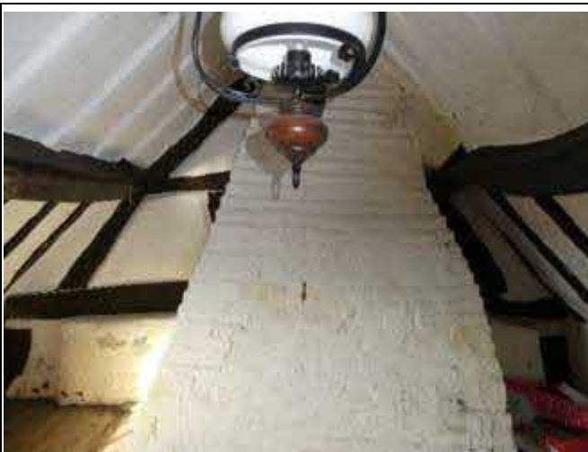
Brick Painted Chimney Breast
