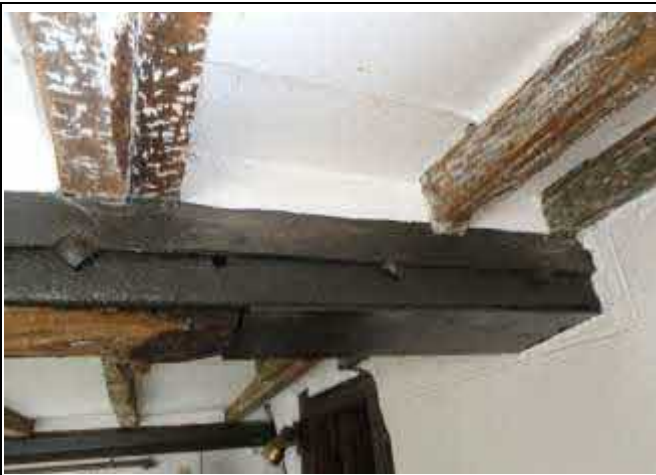
Steel Fortified Central Beam
