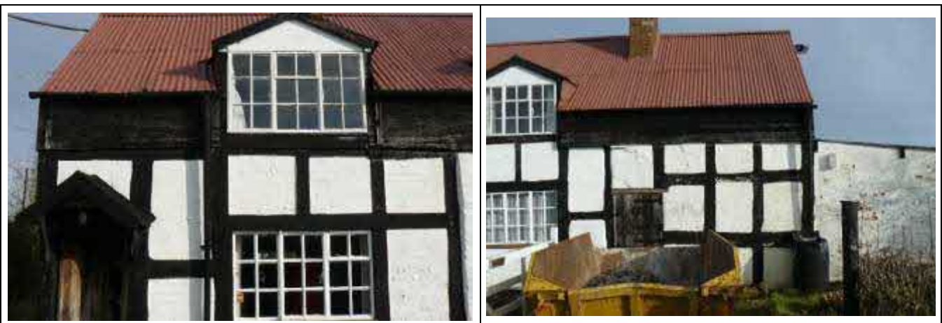
The Primary Façade (South Elevation)
