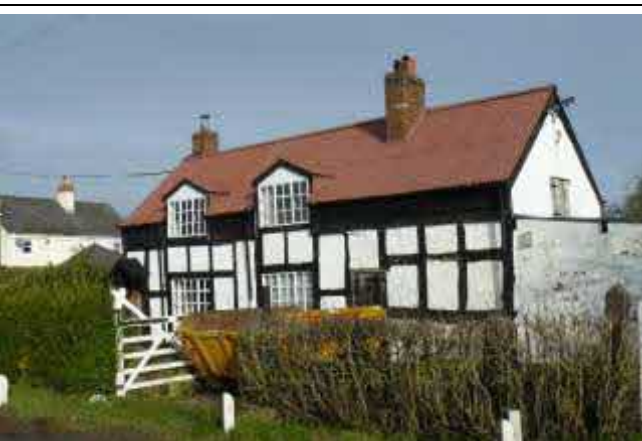
Wooden Gate off Burwardsley Road (South Boundary)
