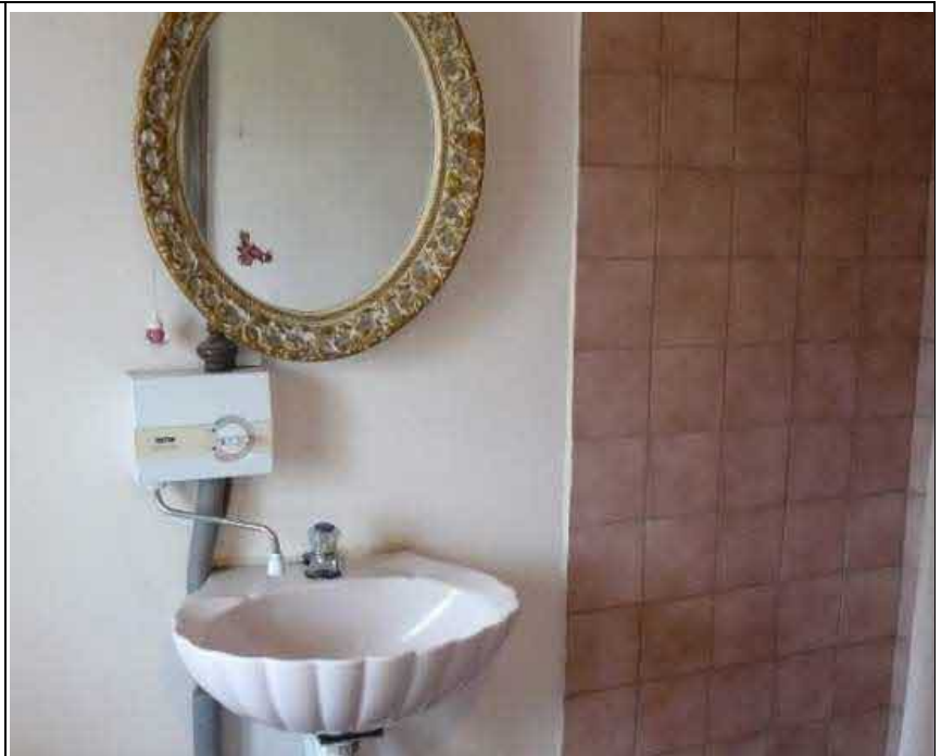
Wash Hand Basin and Tiled Shower Area
