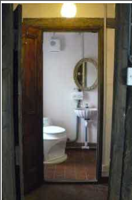
Quarry Tiled Floor
