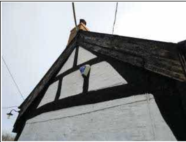
Tiebeam Collar and Truss
