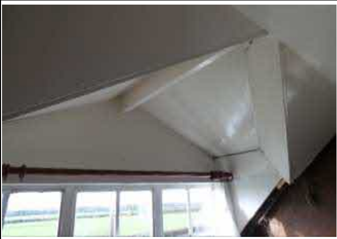
Roof Structure Above Dormer Window
