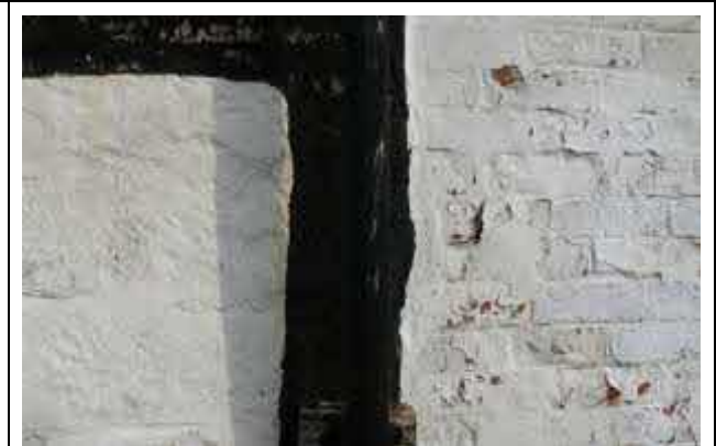
Join Between the Extension and the Garage
