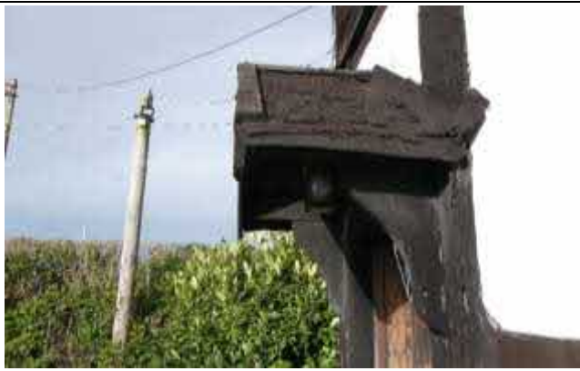
Timber Canopy over Front Door
