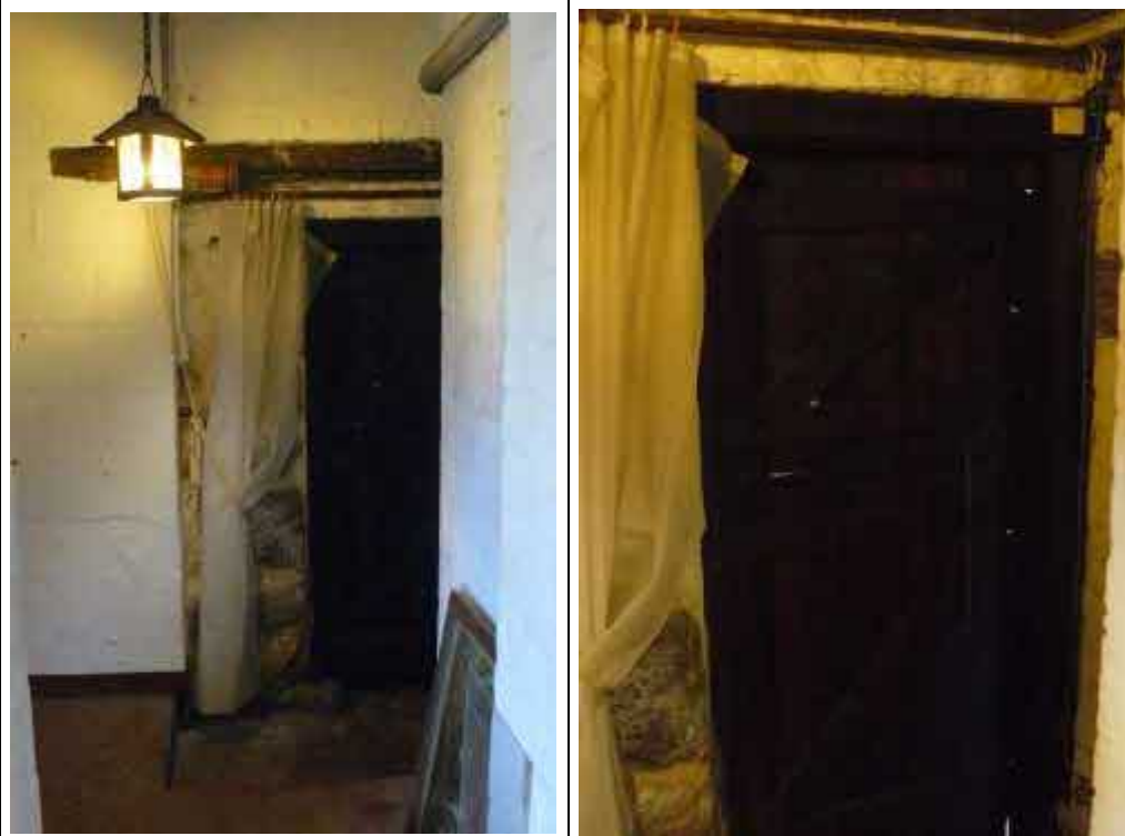
Timber Door to South Wall
