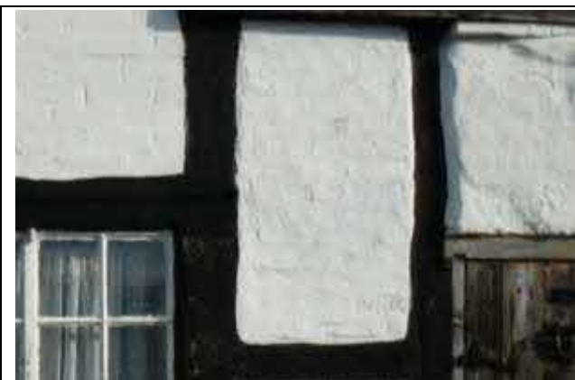
Timber and Paintwork to Replicate Timber
