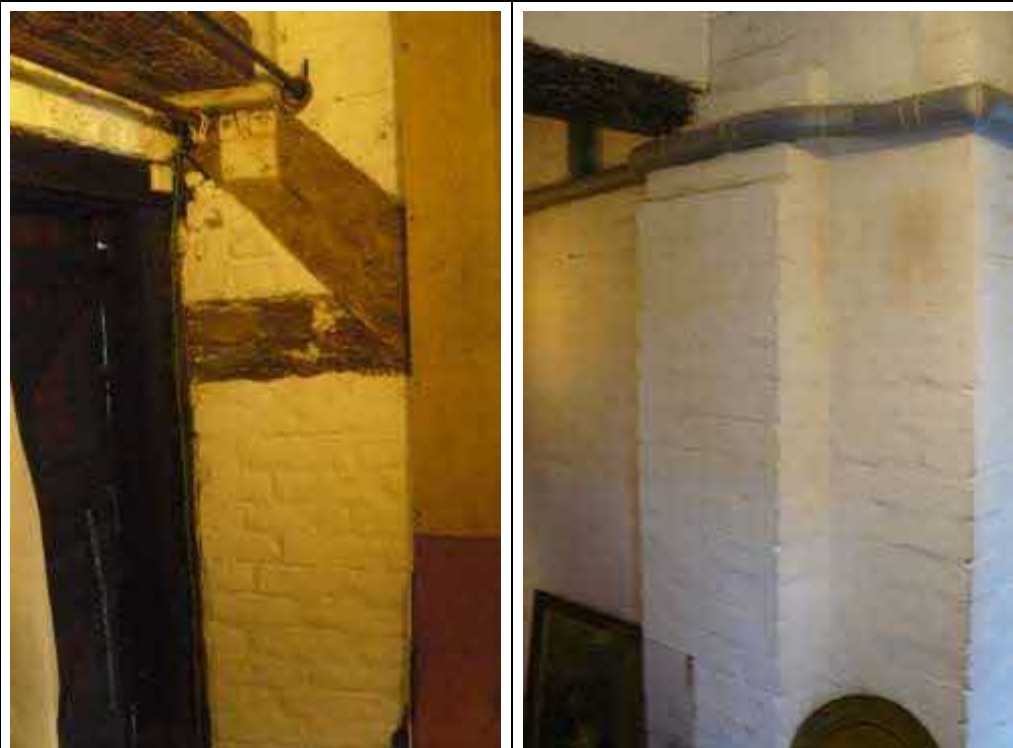
West Wall Showing Timber Frame
