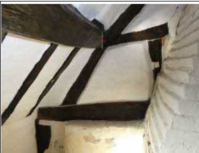
Exposed Tiebeam and Rafter on Either Side of the Chimney Breast
