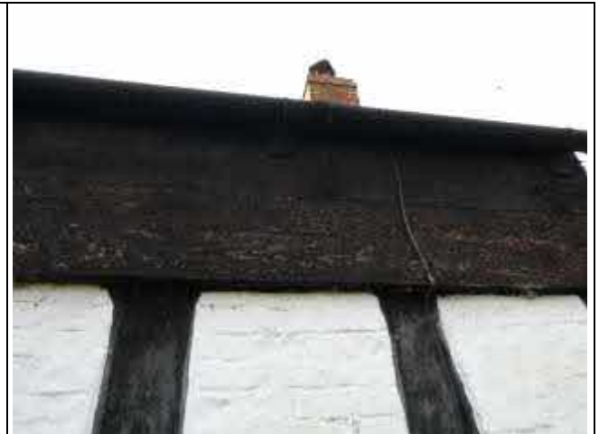
Horizontal Timber Planks
