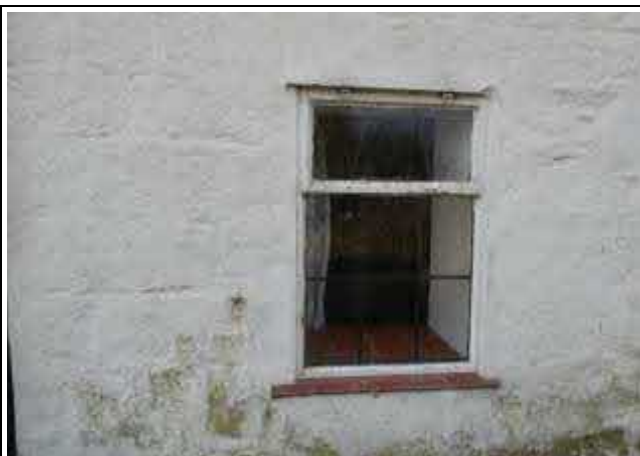
Small Window to East End of the North Elevation
