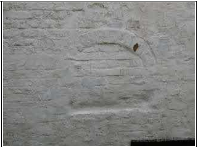
Blocked Brick Oven Arch
