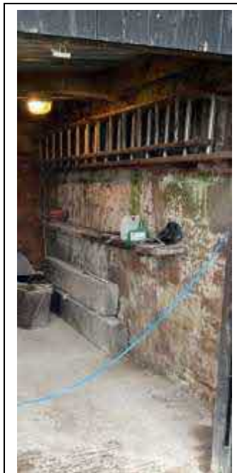
Northeast Internal Wall to Garage
