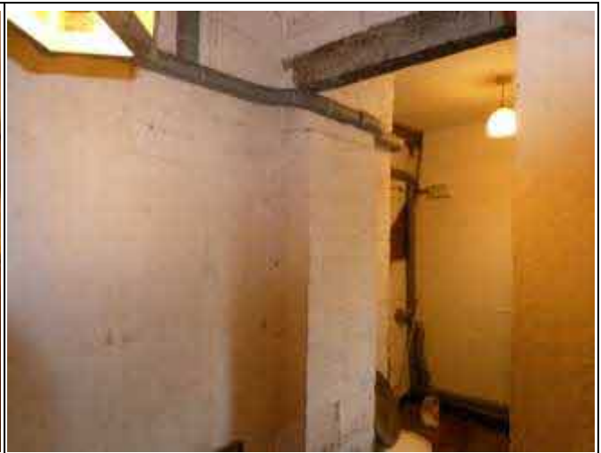
Metal Pipe on the South Wall
