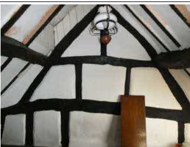
Timbered Gable Wall
