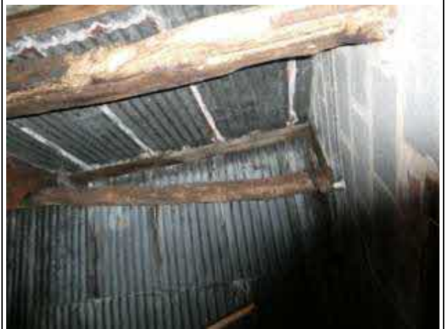
Timber Beams Supporting Metal Corrugated Roof
