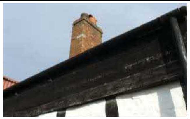
Timber Planks Covering the Thatched Roof
