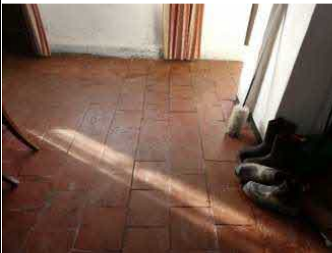
Quarry Tiled Floor
