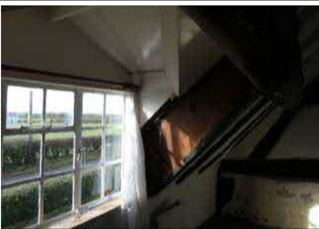
Window to the South Wall
