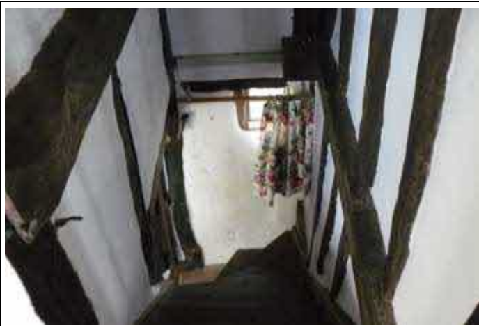
Timber Framed Walled Stairwell
