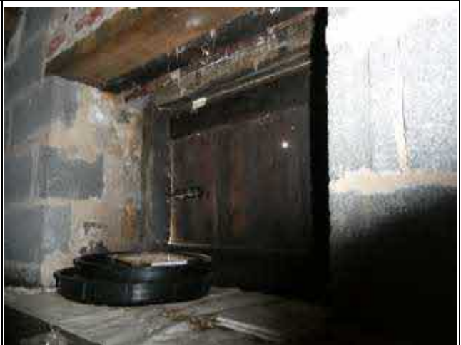
Timber Door at the East Wall
