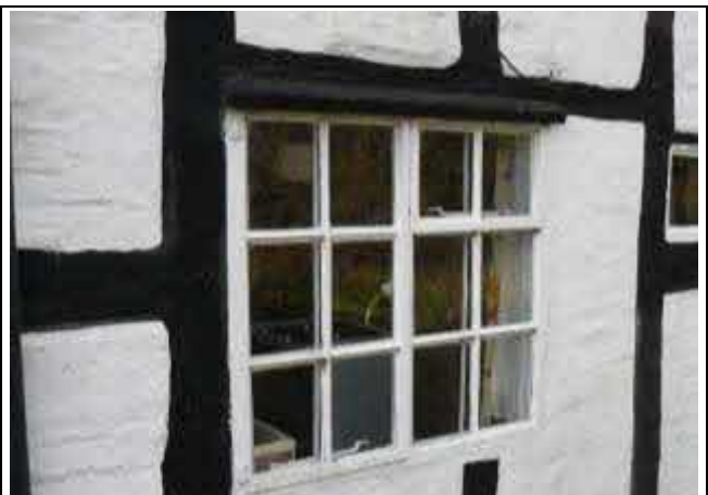
Central Window to East Elevation
