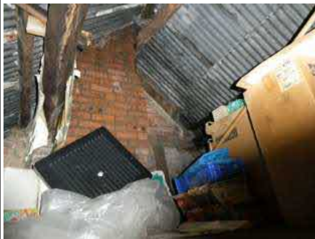
Chimney Breast and Timber Frame at the West Wall
