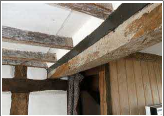
Steel Fortified Central Beam
