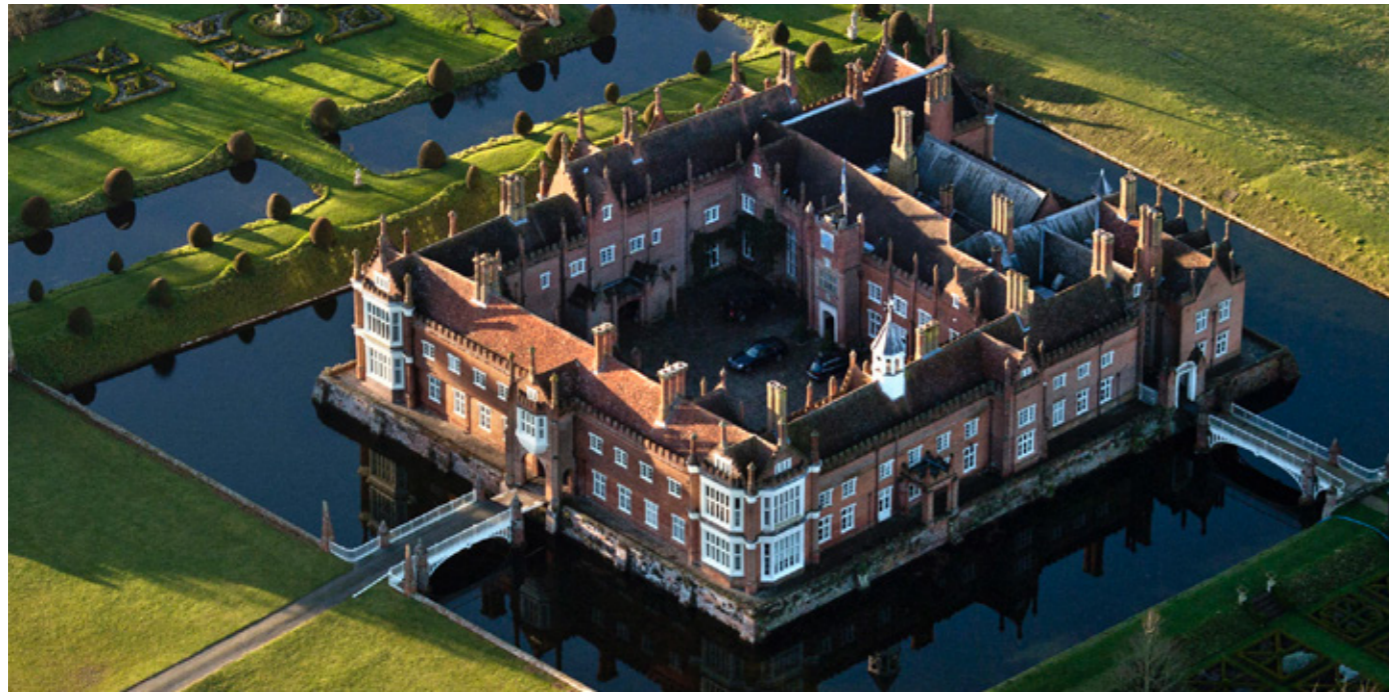
Fig. 19 Aerial view of the hall from the south-east.
