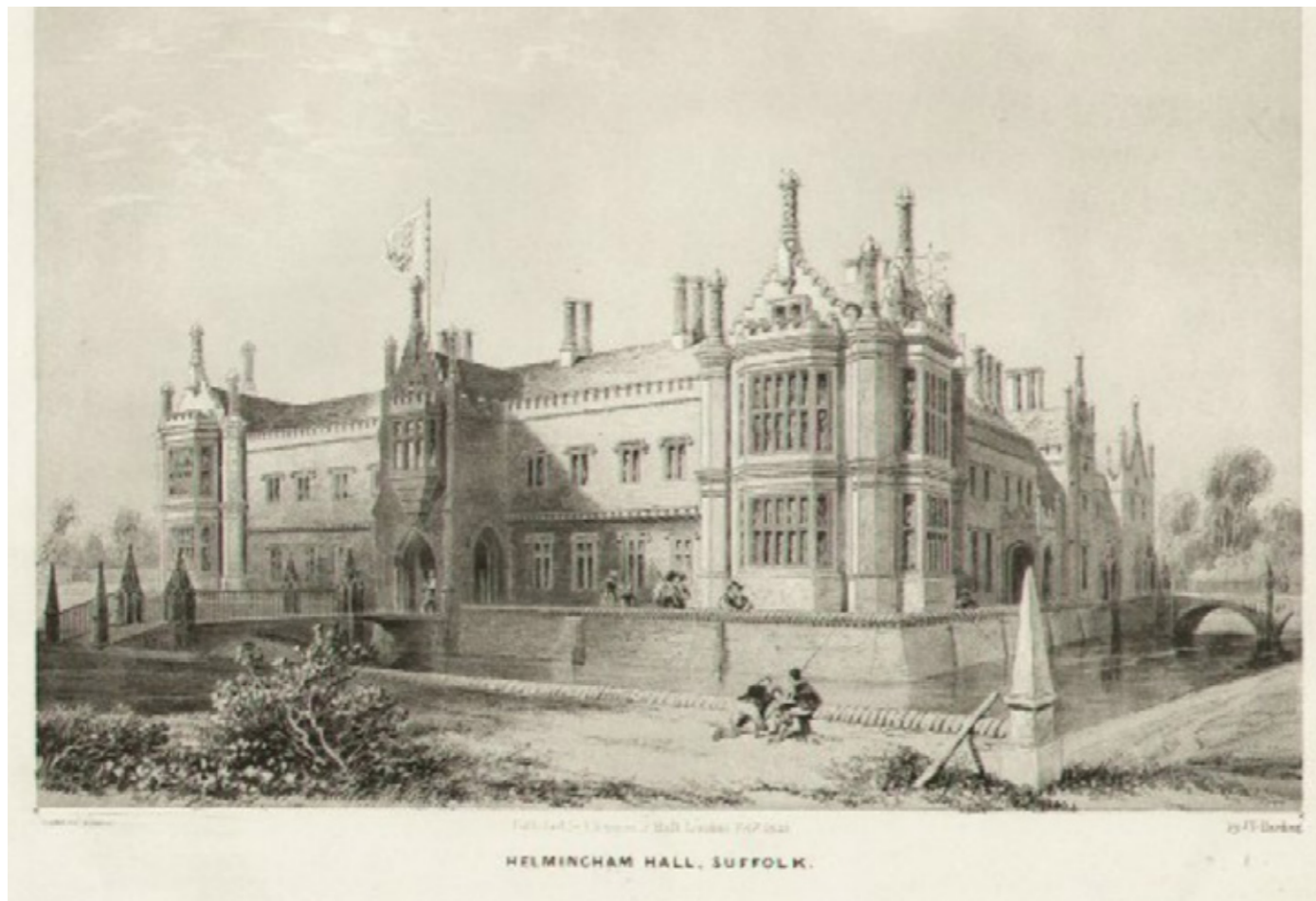
Fig. 11 View of South front, between 1800 - 1840 showing Nash's rendered finish.
