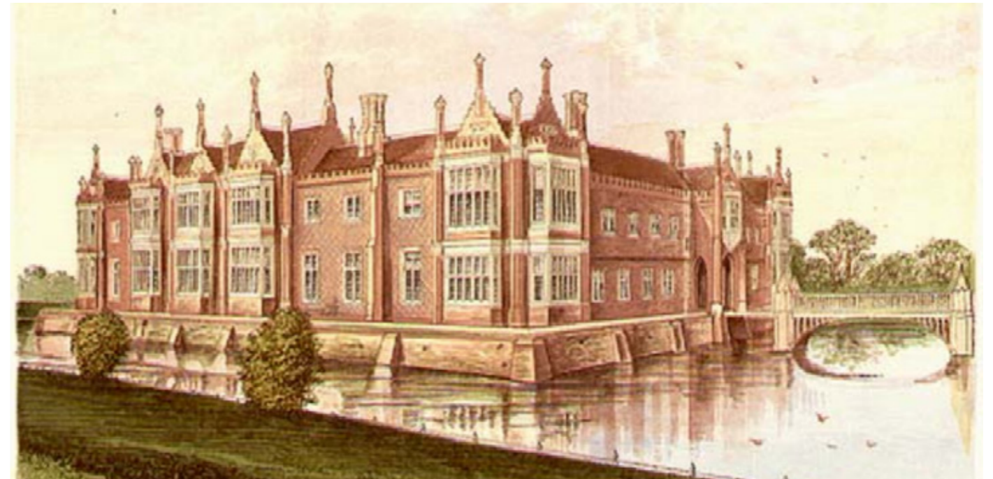
Fig. 17 View of the west front as refaced by Salvin in 1840's. Salvin rebuilt the north end to create a generous Victorian dining room, drawing room and staircase hall. The rest of the facade was refaced and two storey bay windows were added.
