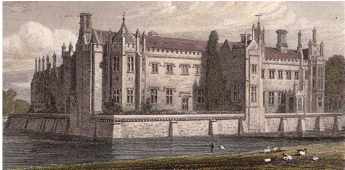
Fig. 15 c. 1810 view of the west front showing Nash's alterations along with the grey render resigned to imitate rubble stone
