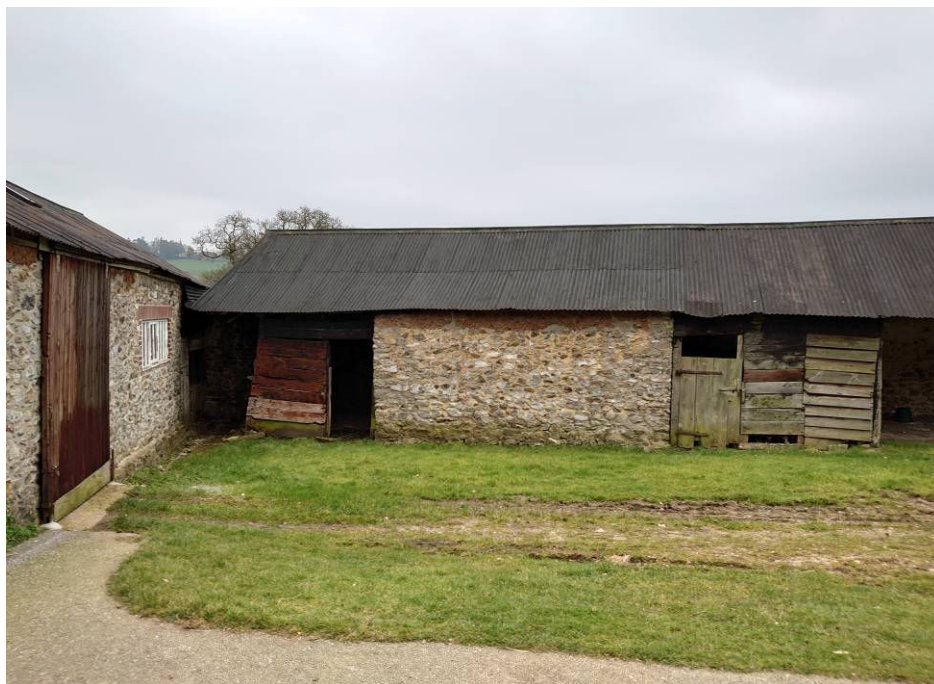
Figure 8. Yard elevation of Barn 2
