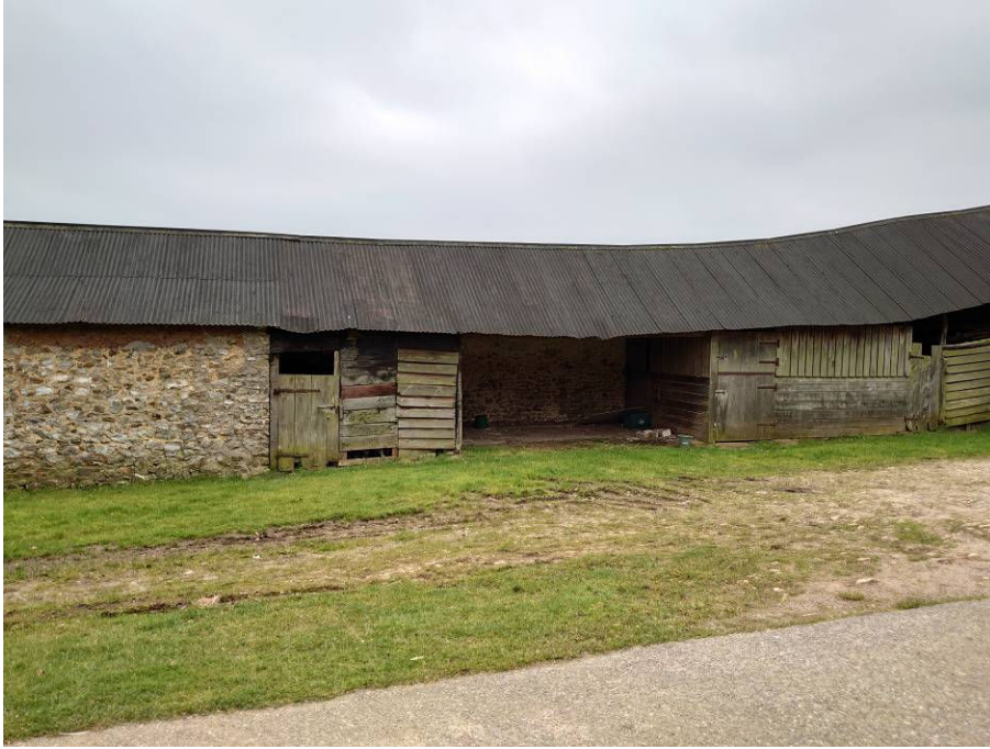
Figure 9. Yard elevation of Barn 3
