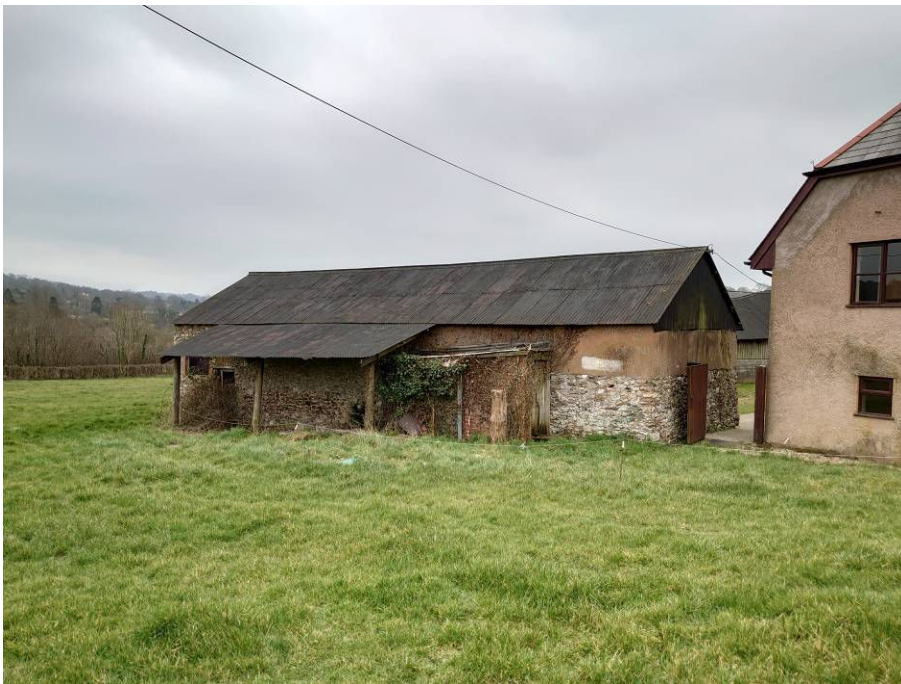
Figure 10 rear elevatio of barn 1
