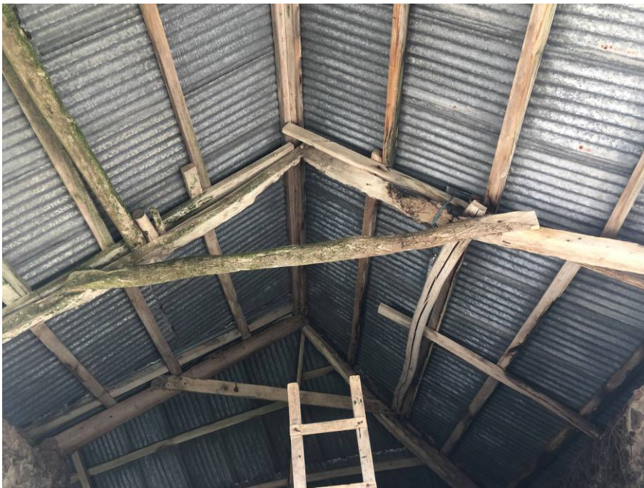
Figure 6. Roof over barn 5 showing structure
