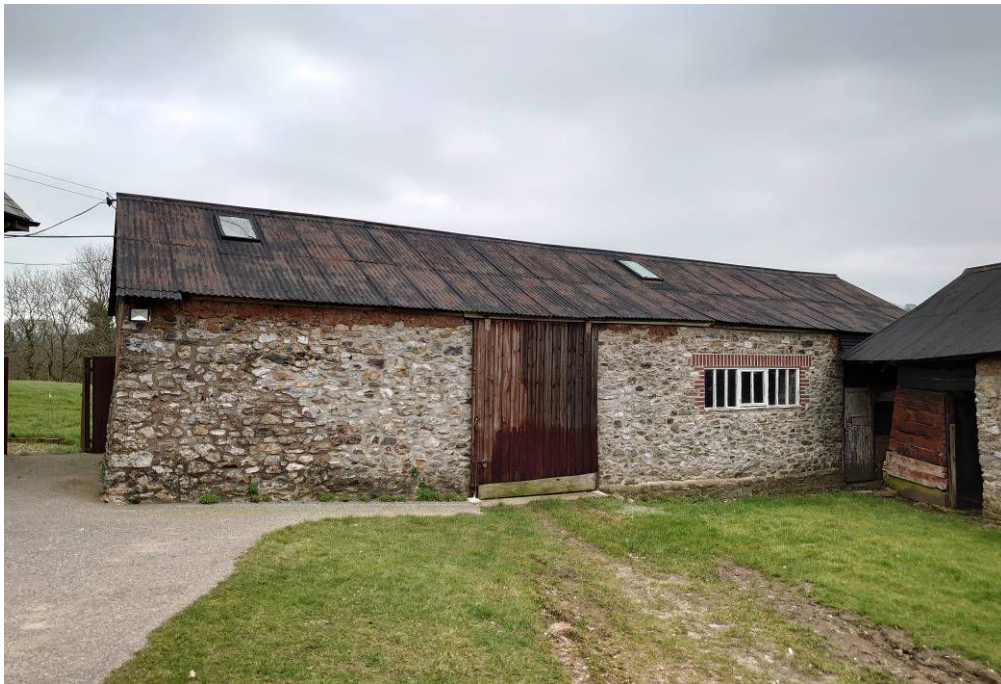
Figure 7 Yard elevation of threshing barn.
