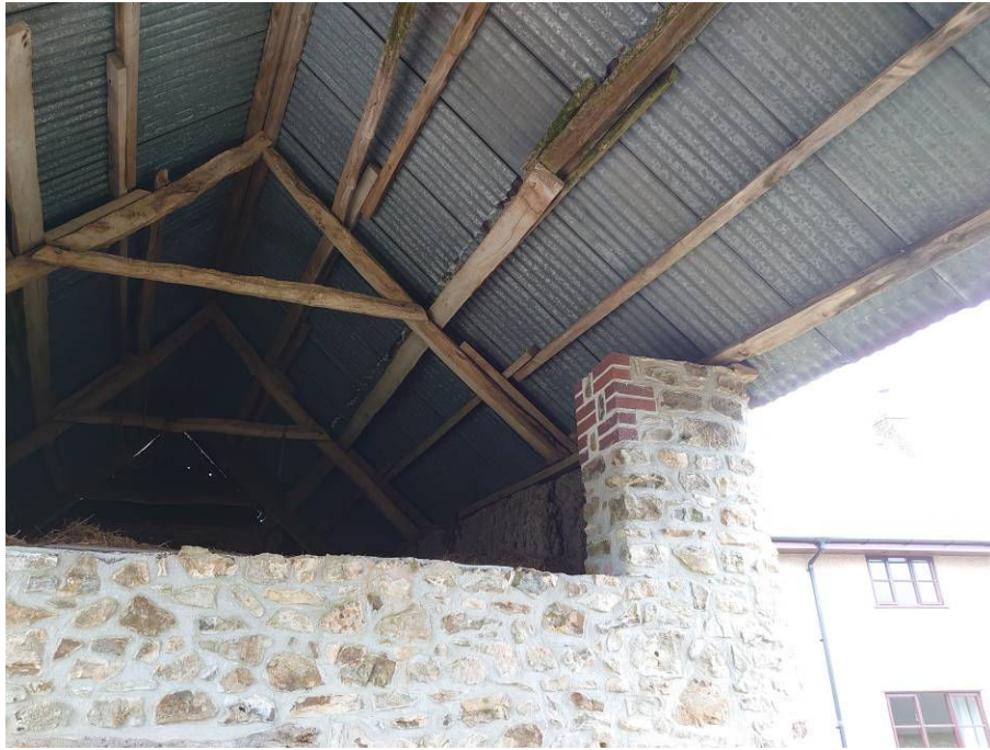
Figure 5 Roof over Barn 6
