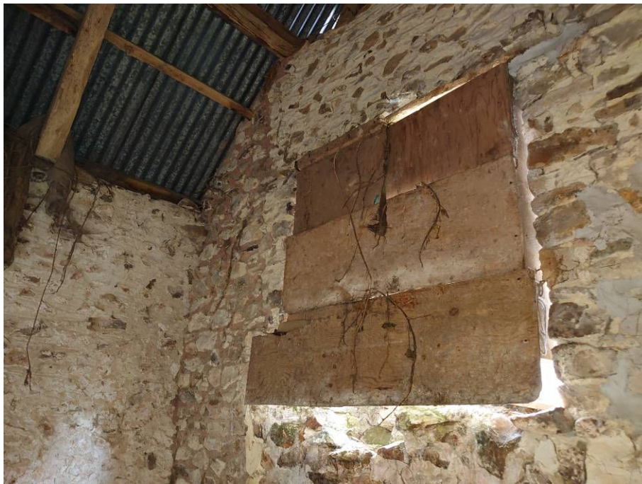
Figure 122. Internal of end elevation of Barn 6
