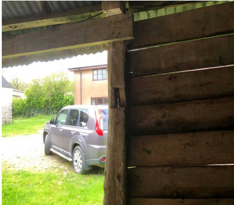
Figure 2 showing Linhay post with mortise hole.
