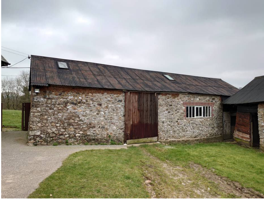
Figure 1 Threshing barn and part of cobbled yard
