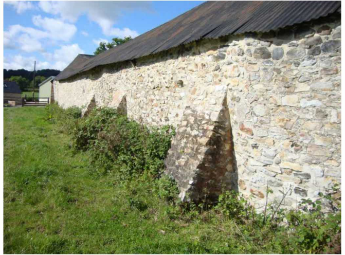
Photo 10- South Eastern Wall
