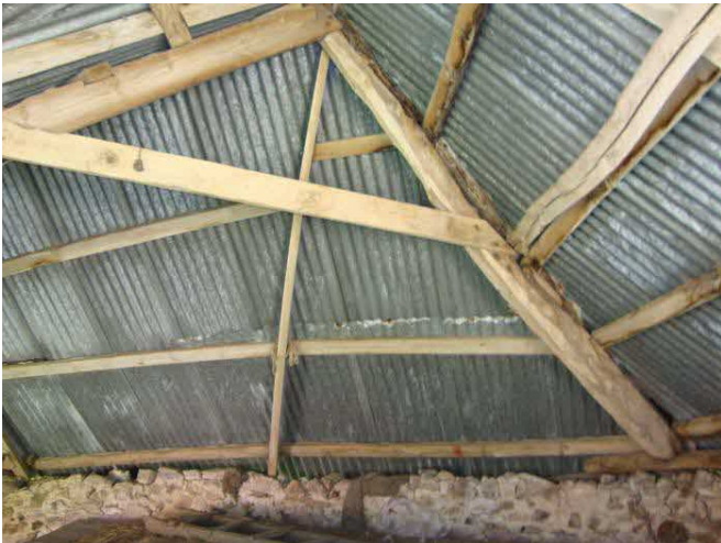
Photo 7 –South Corner Roof
