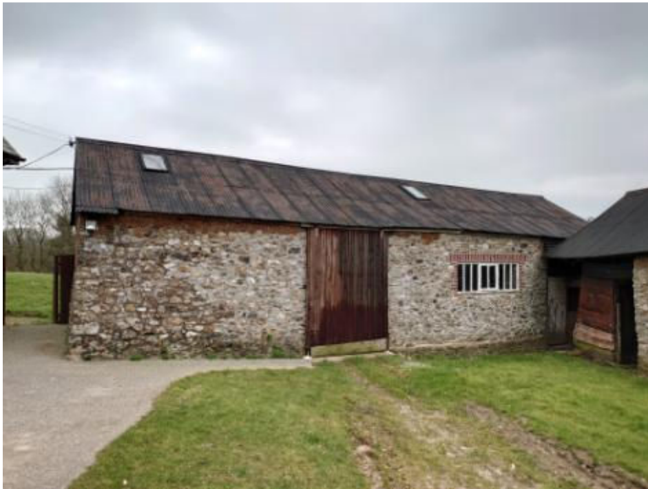
Fig.3 – Site Photo – View of NE barn from within courtyard.
