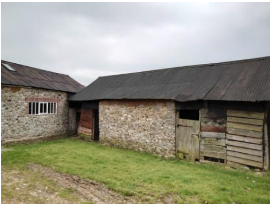
Fig.2 – Site Photo – View of East corner of courtyard.
