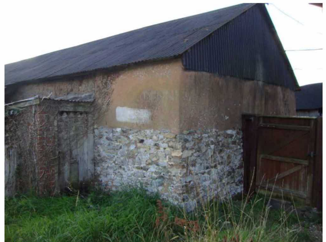
Photo 12 – North Western Wall
