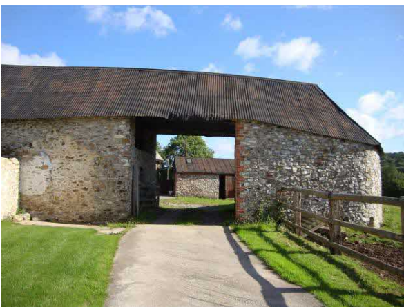
Photo 1 –Side View –South West
