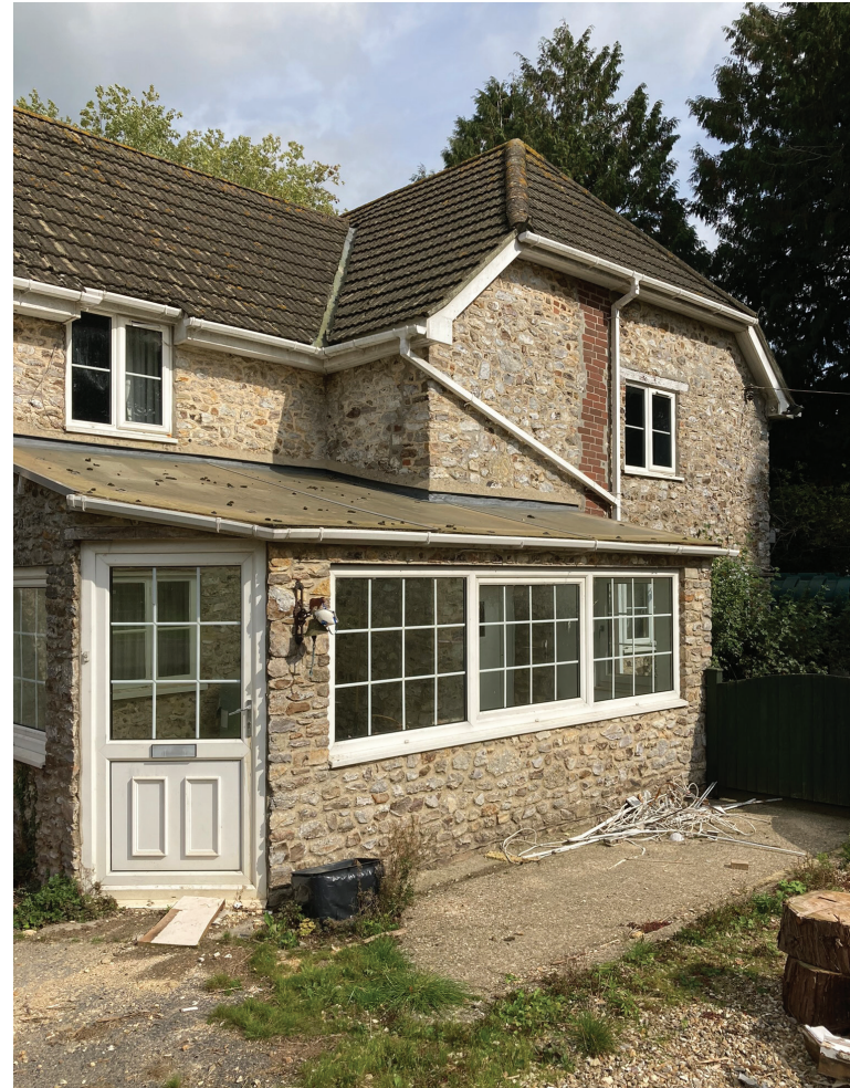
Figure 7 - Front view of the property
