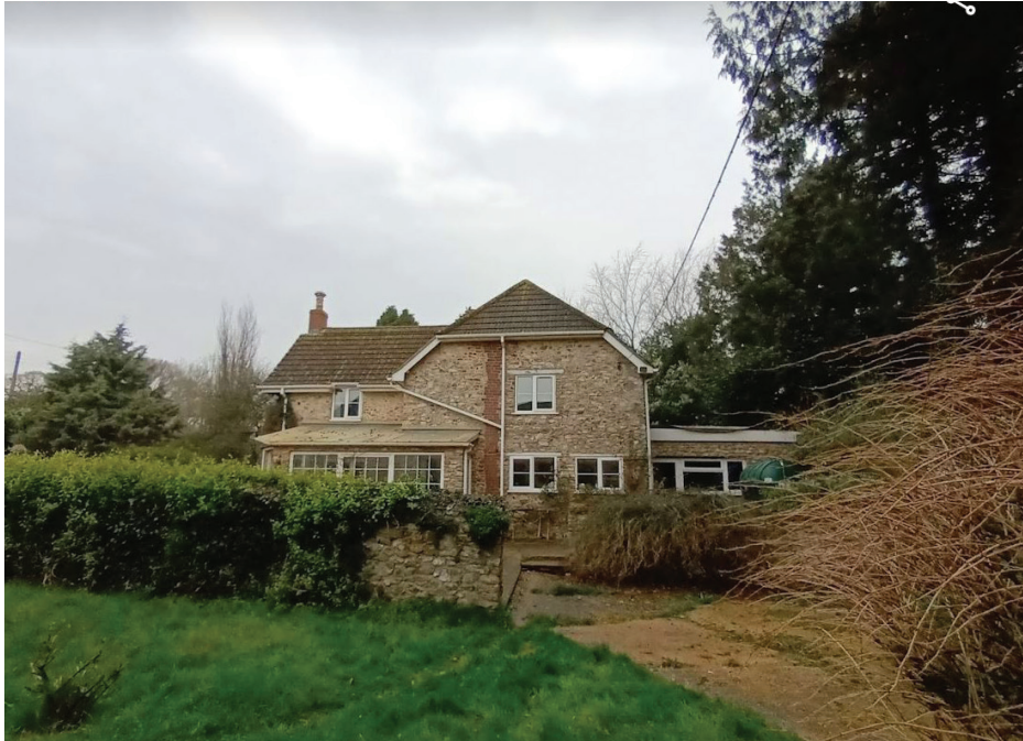
Figure 8 - Front view of the property
