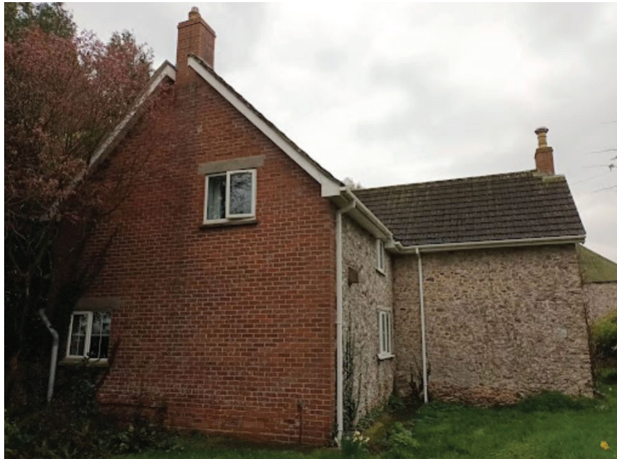
Figure 10 - Rear view from the north west
