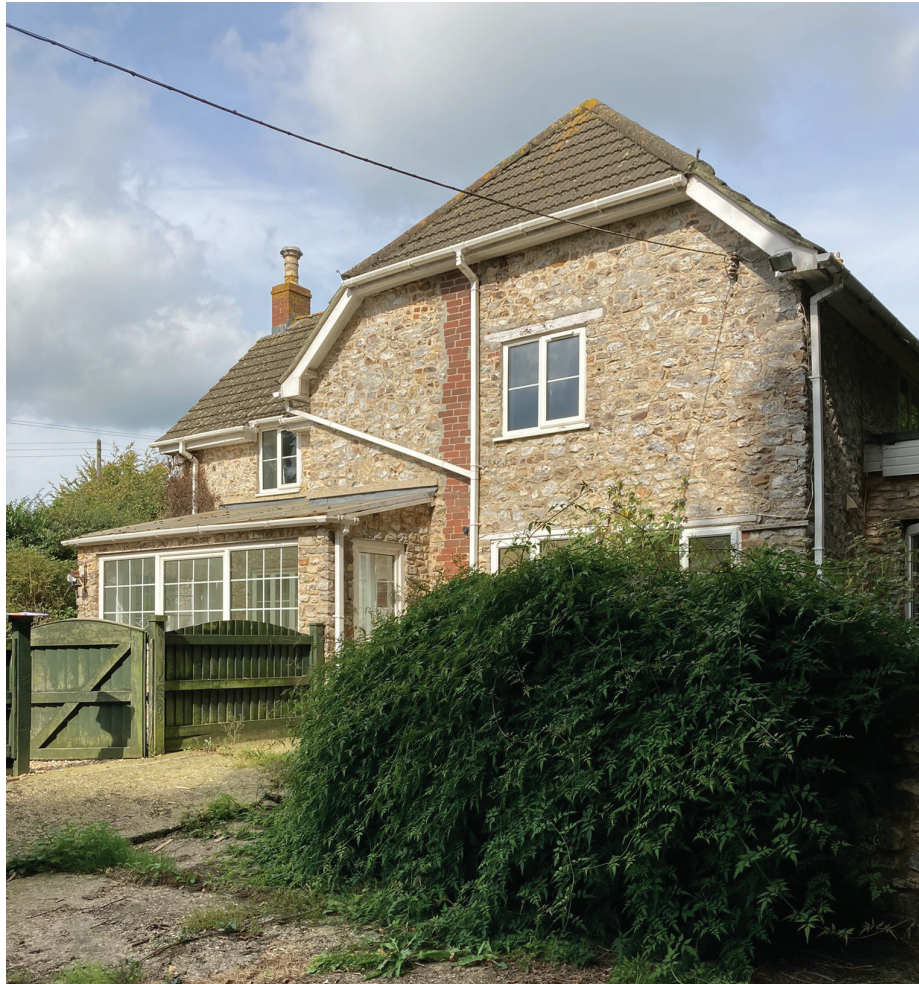
Figure 6 - Front view of the property
