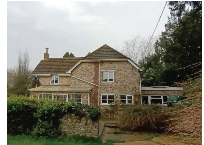
Figure 3 - Front view of existing dwelling
