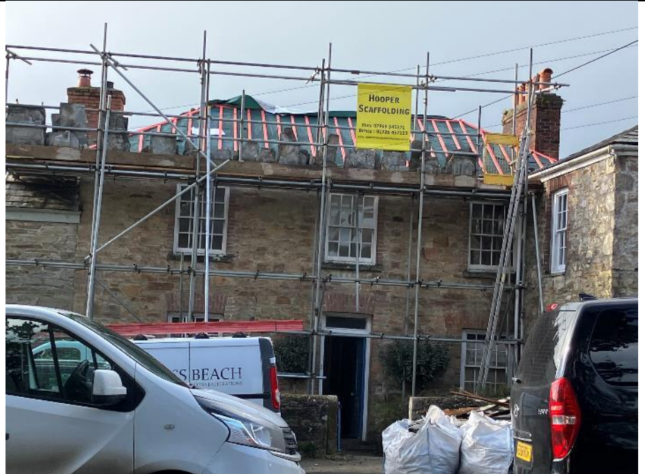
Photo 1: Showing the front elevation of the building.
