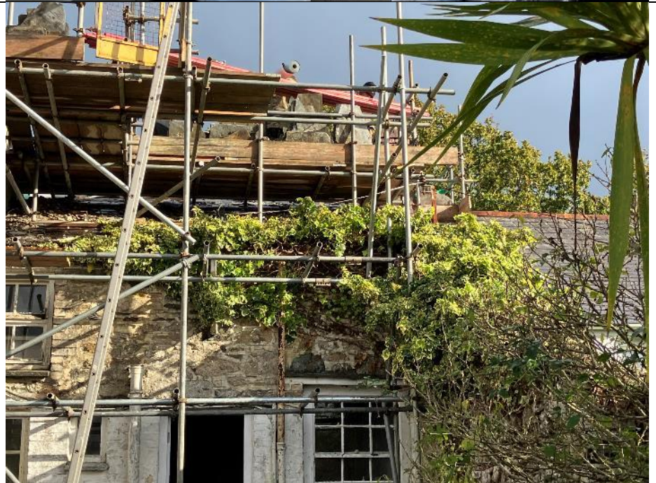
Photo 2: Showing the extension at the rear elevation of the building. Although some tiles remained on this elevation, they were tight fitting and no gaps were identified in which bats or birds could access the building.
