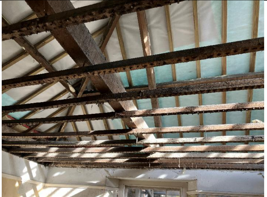
Photo 5: Showing the roof exposed from all elevations.
