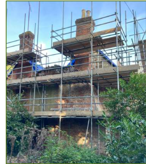
East and west elevation after the removal of the cementitious render.
