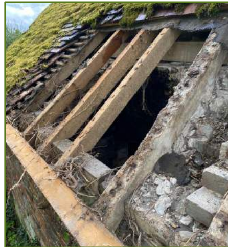
Location of proposed metal flue and chimney gather.
