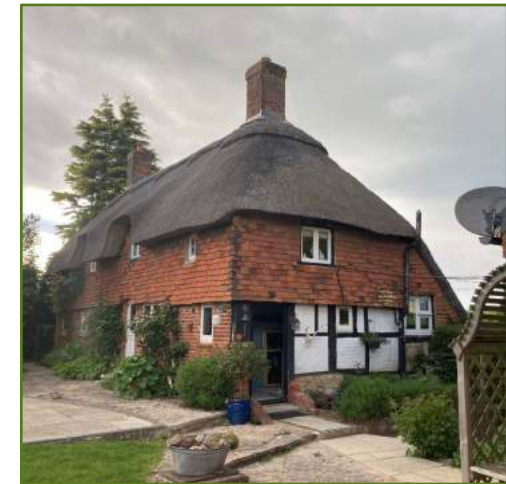
Tile hanging proposed to gable ends (left) and example of traditional tile hanging in a timber-framed cottage in Binsted (Hampshire).
