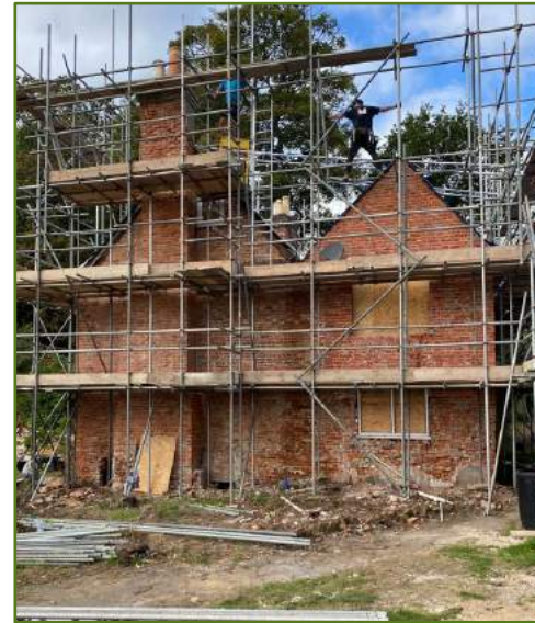
East and west elevation after the removal of the cementitious render.
