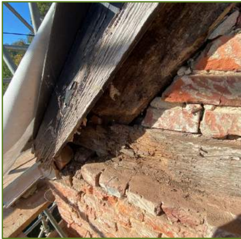
Eastern chimney stack to be rebuilt and reattached (top) and original frame's joints to be strapped (bottom).
