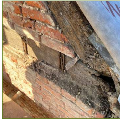
Eastern chimney stack to be rebuilt and reattached (top) and original frame's joints to be strapped (bottom).
