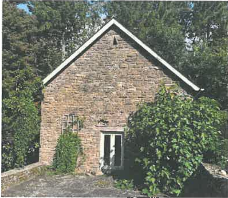
Photo of the south elevation of the outbuilding
