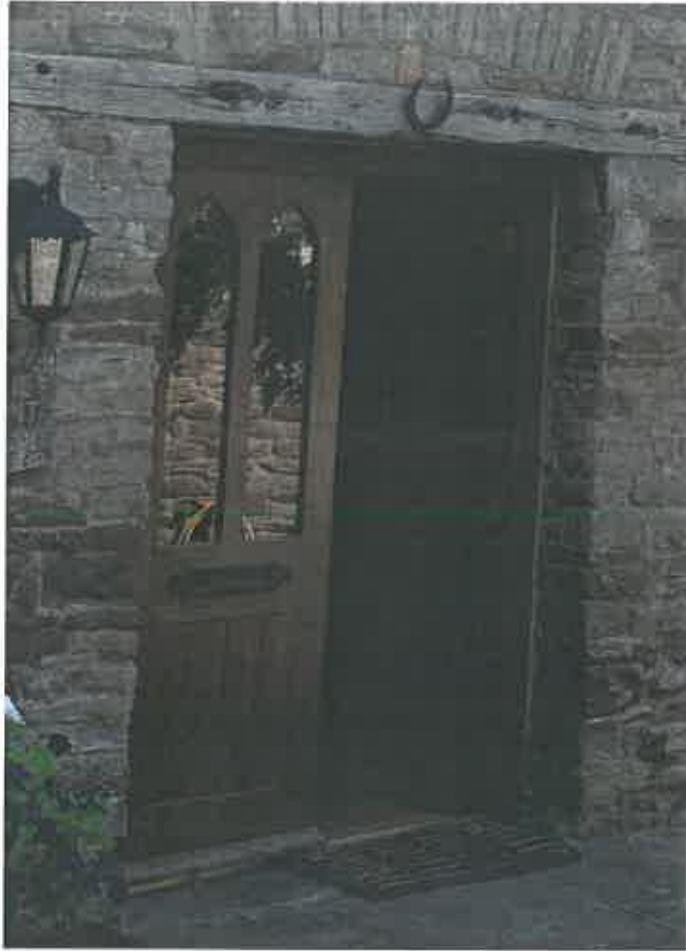
Existing front door with smoke glazing
