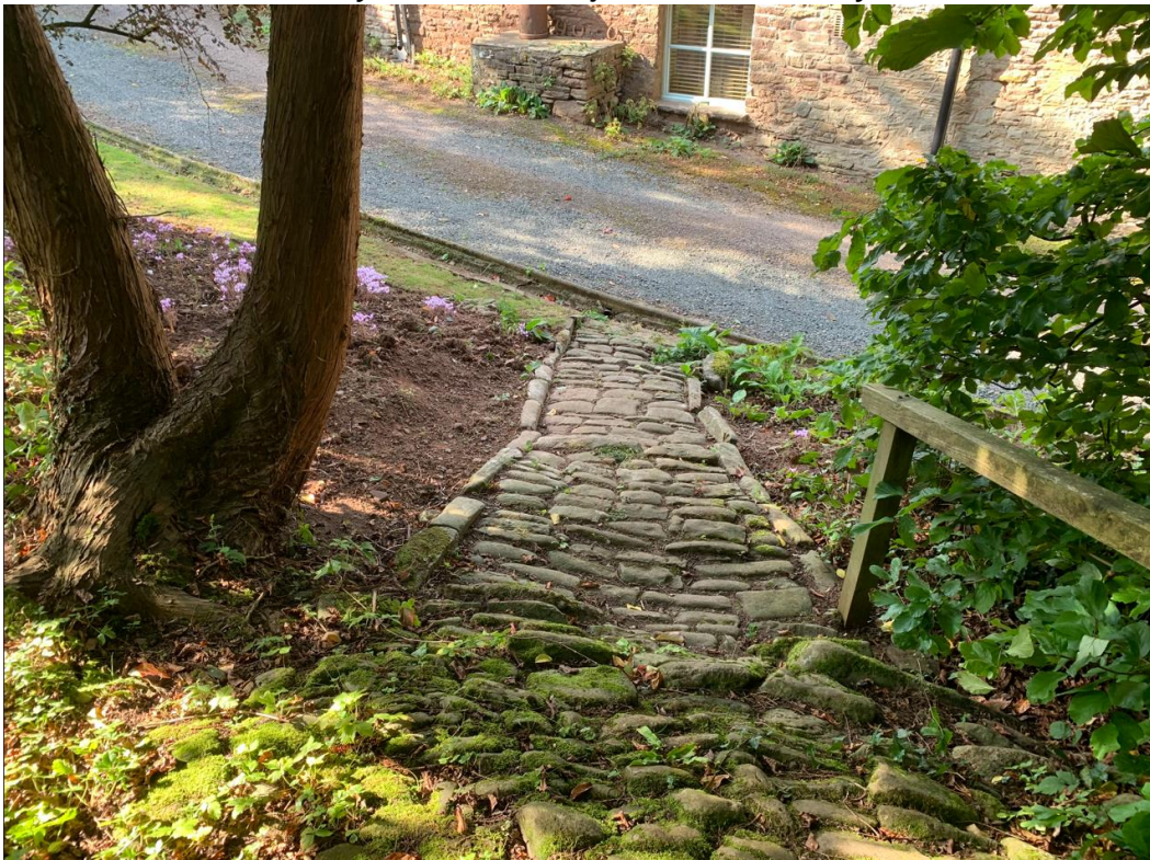
View of the cobbles from the little barn showing the uneven nature
