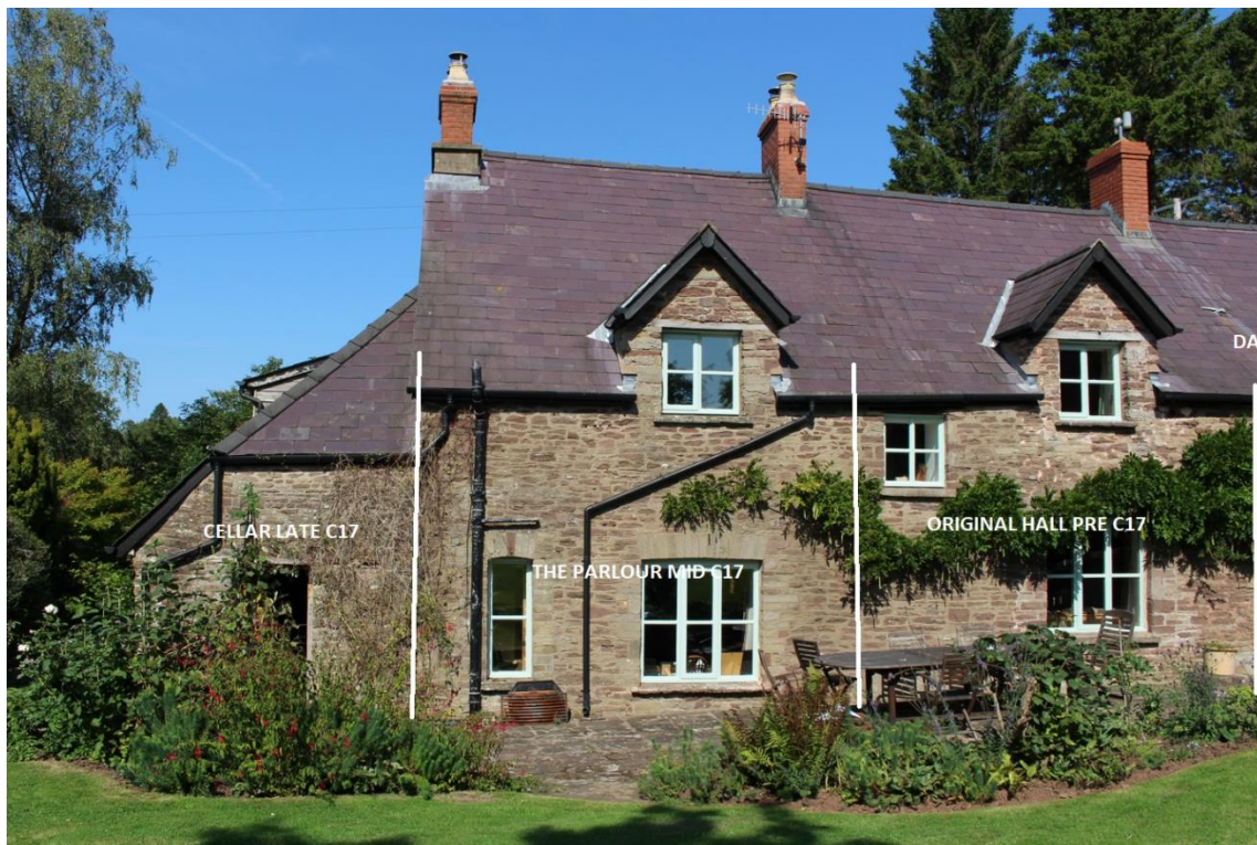
Photo of the south elevation with the phased development indicated
