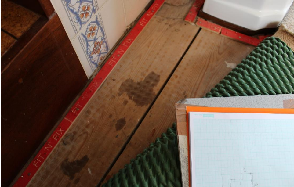
Softwood floorboard in the bathroom
