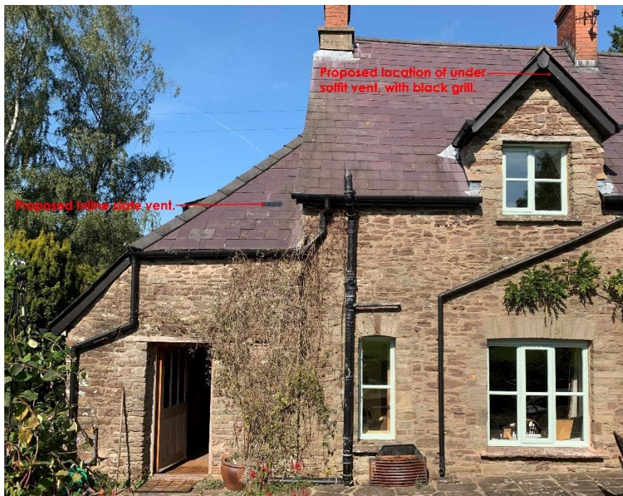
Inline slate vent in roof of cellar
