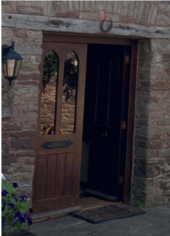
Existing front door with smoke glazing
