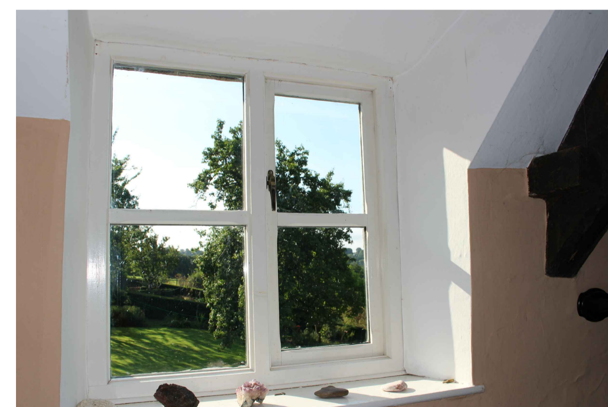
WINDOW WITH SLOPING SOFIT OVER
