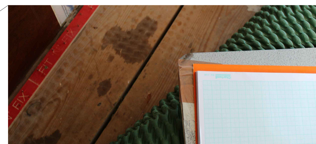
EXISTING MODERN FLOOR BOARDS
