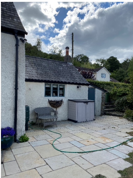
Location for the kitchen extension on the north west gable end
