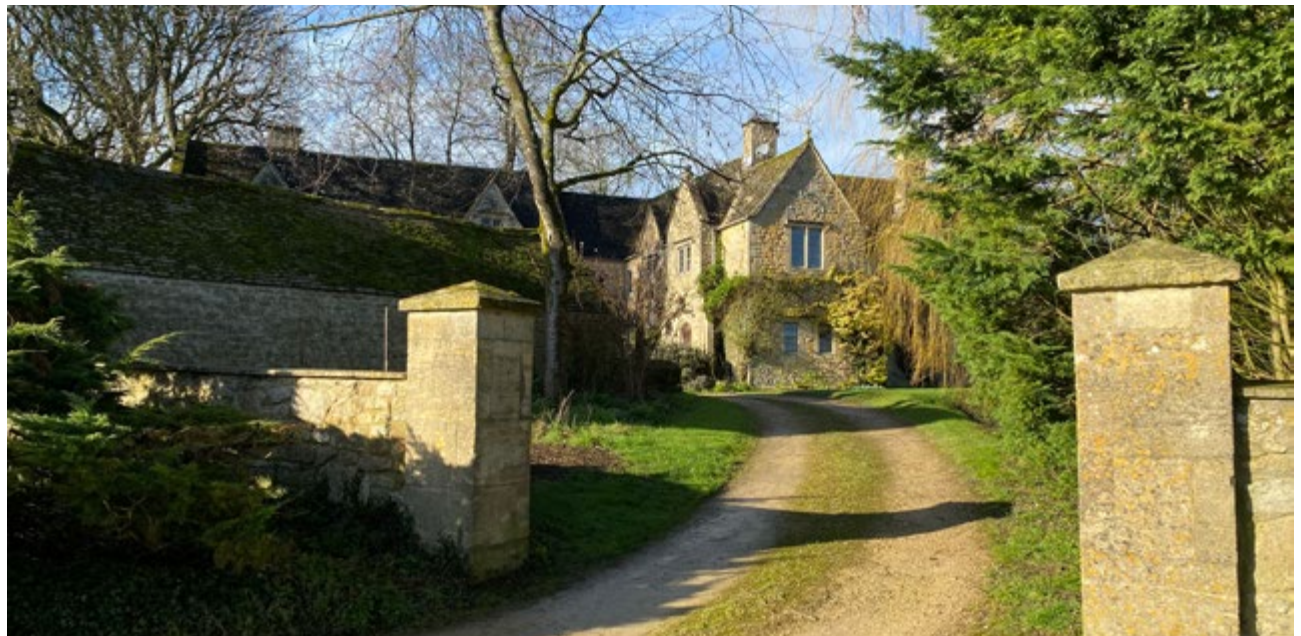
The Dower House - Grade II listed
