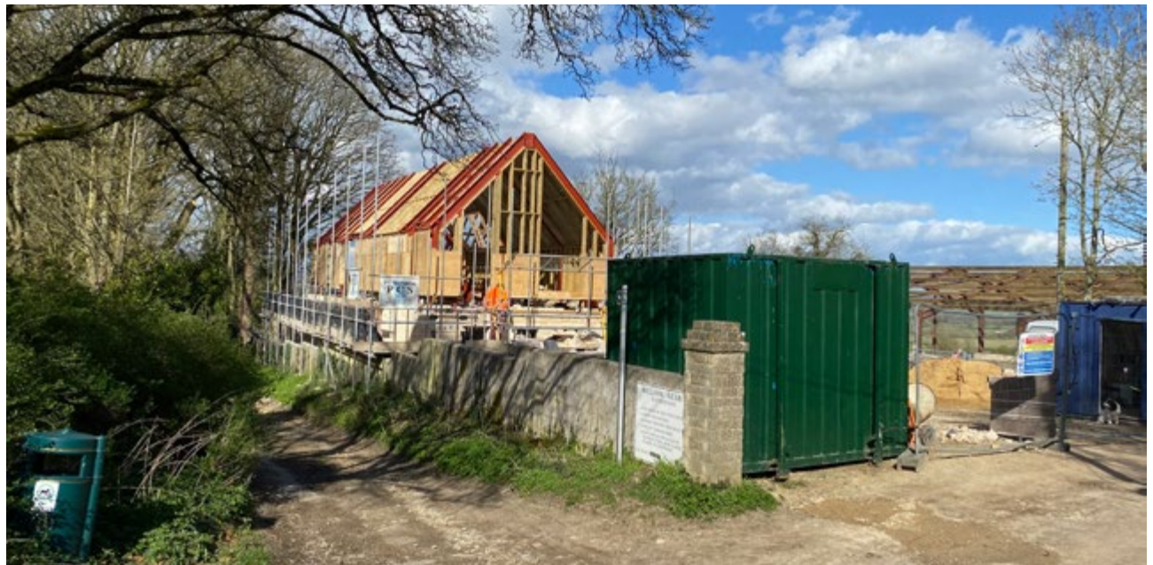
Wallground new dwelling in progress app. ref.:19/03873/FUL
