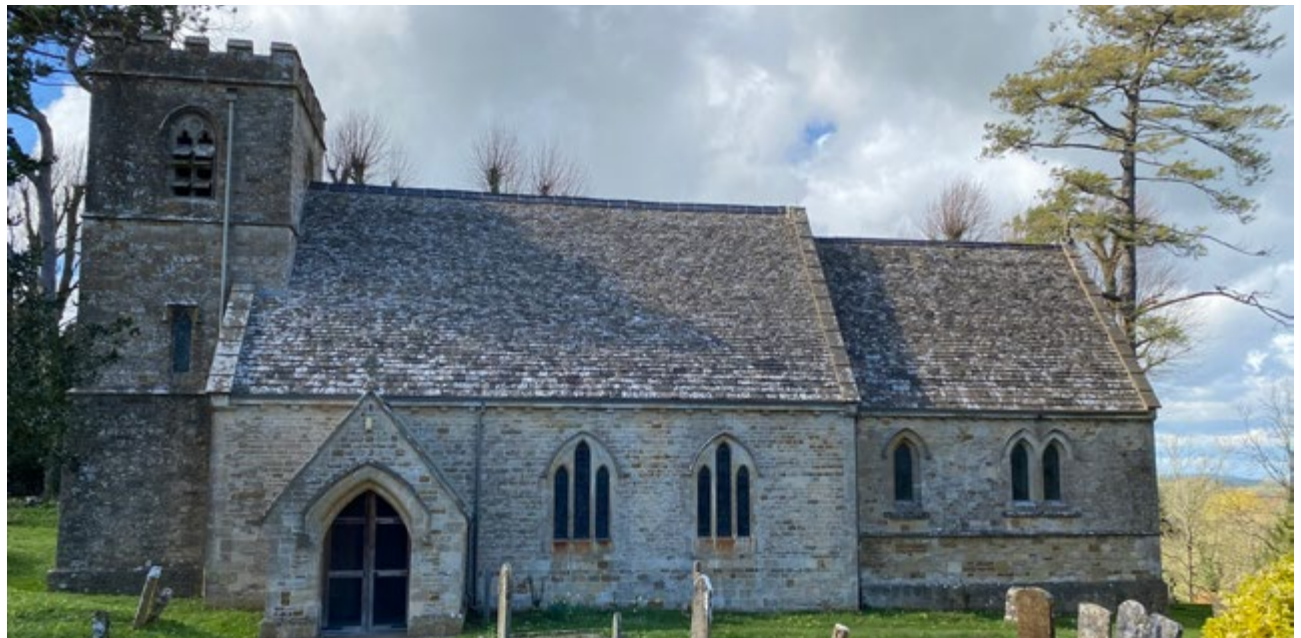
St Mary's Church - Grade II listed
