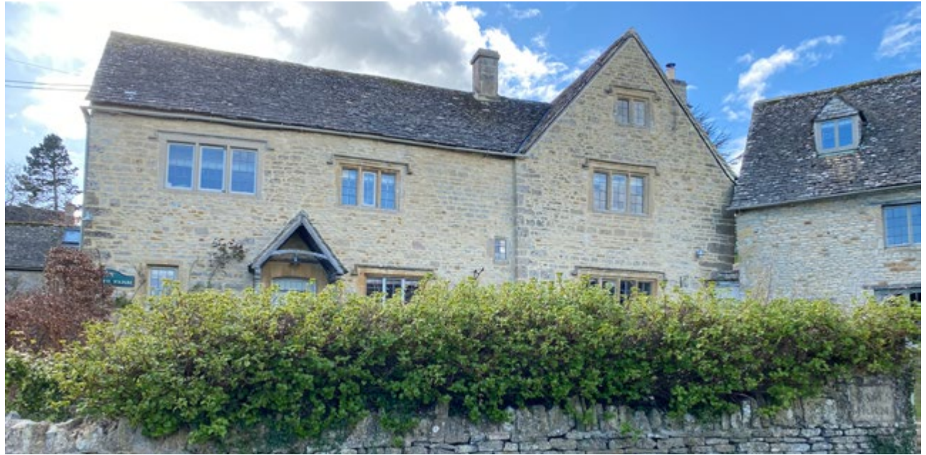
Stayts House - Grade II listed
