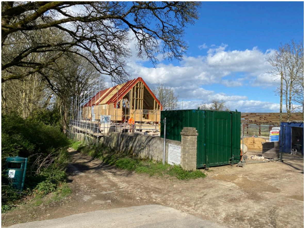
19/03873/FUL - Photo of application site with building in progress
