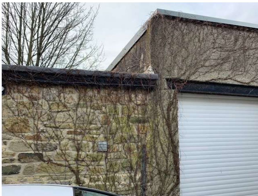
East Elevation at abutment to Cragdale Garage
