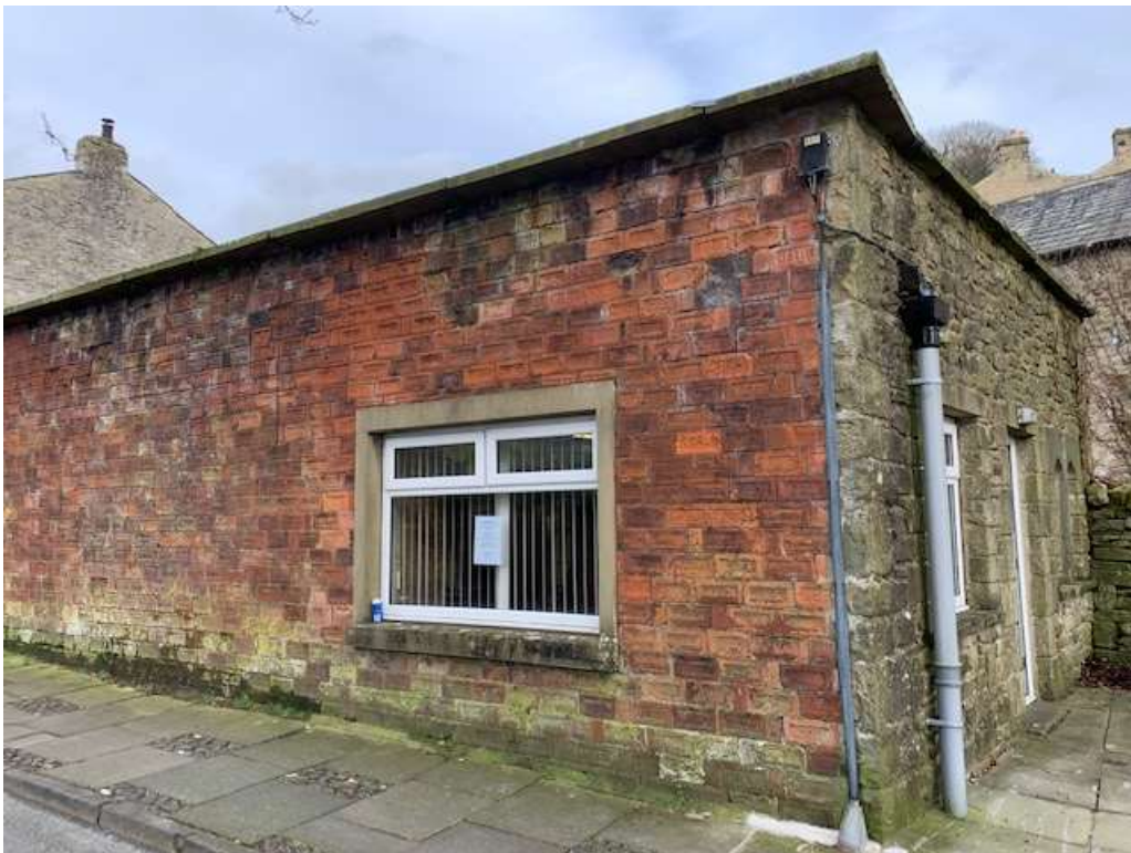
West Elevation faced with brickwork laid on sides
