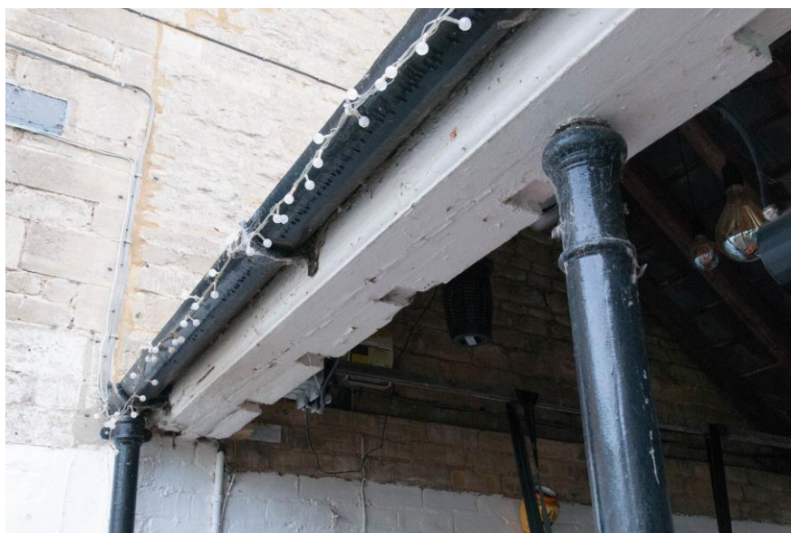
Figure 24 Detail of cast iron column supporting a re-used beam
