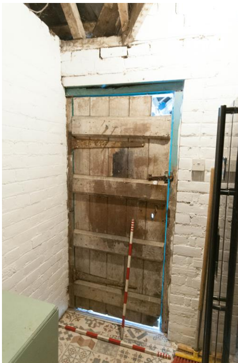
Figure 32 Detail of plank and ledge door to the utility room
