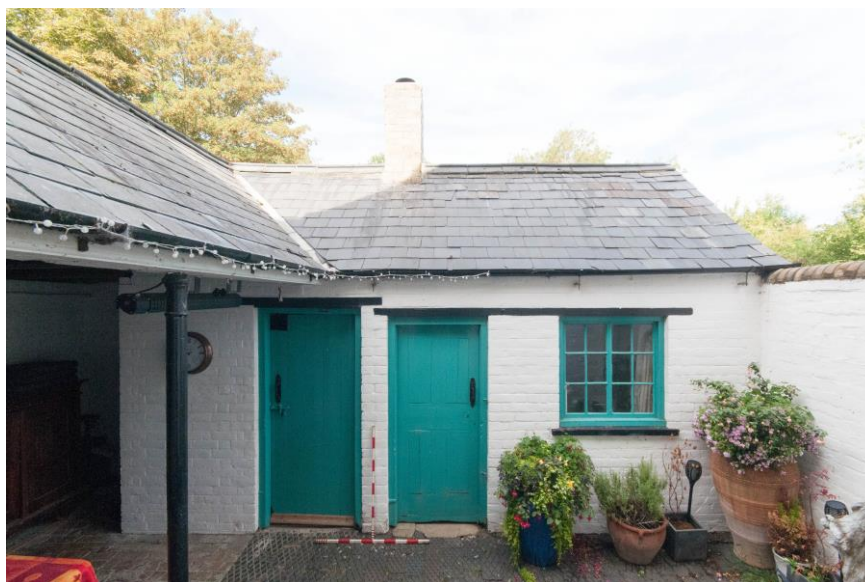
Figure 30 View of the north range, looking north
