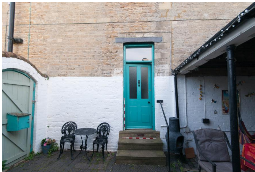
Figure 23 Stepped entrance to the Hall. Note adjacent join to extension
