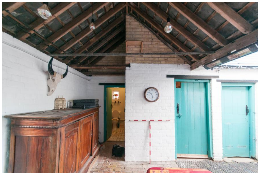
Figure 27 The west range, looking south
