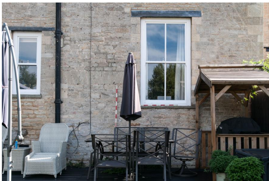
Figure 20 Detail of blocked door with visible lintel adjacent to later sash window
