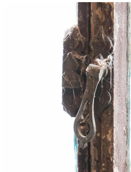
Figure 39 Detail of window latch
