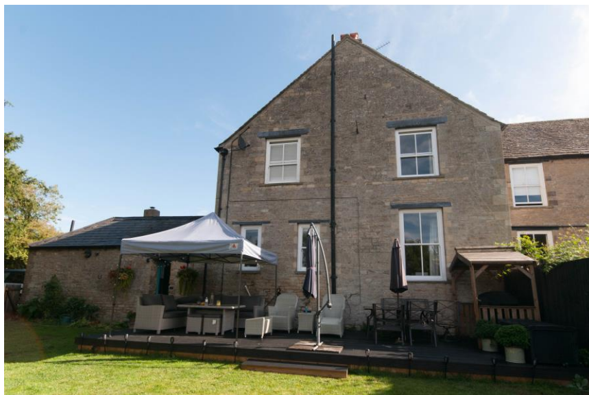
Figure 19 The northern extension, looking east
