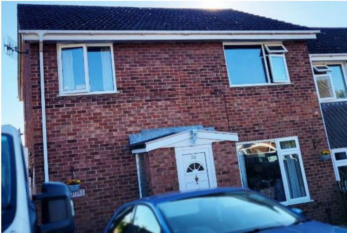
Photograph 1. Exterior. Northeast elevation.
