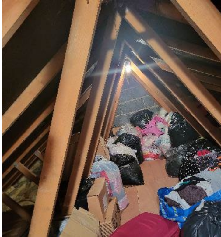
Photograph 3. Interior. View of part of the roof-space. Looking southeast from northwest.
