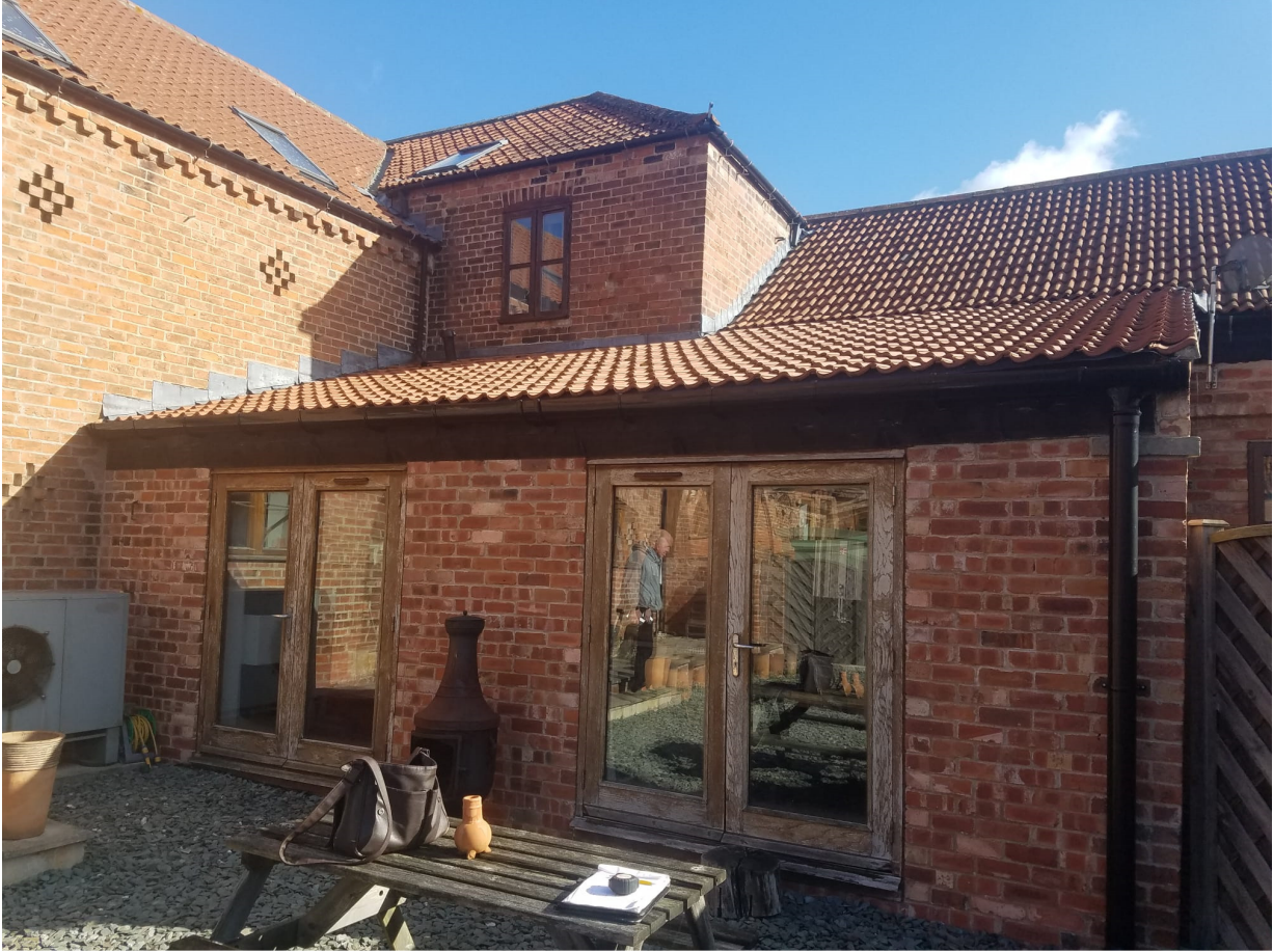
Photograph 2 Showing Existing Front Elevation to Sun Lounge – 3 Prebendary Farm
