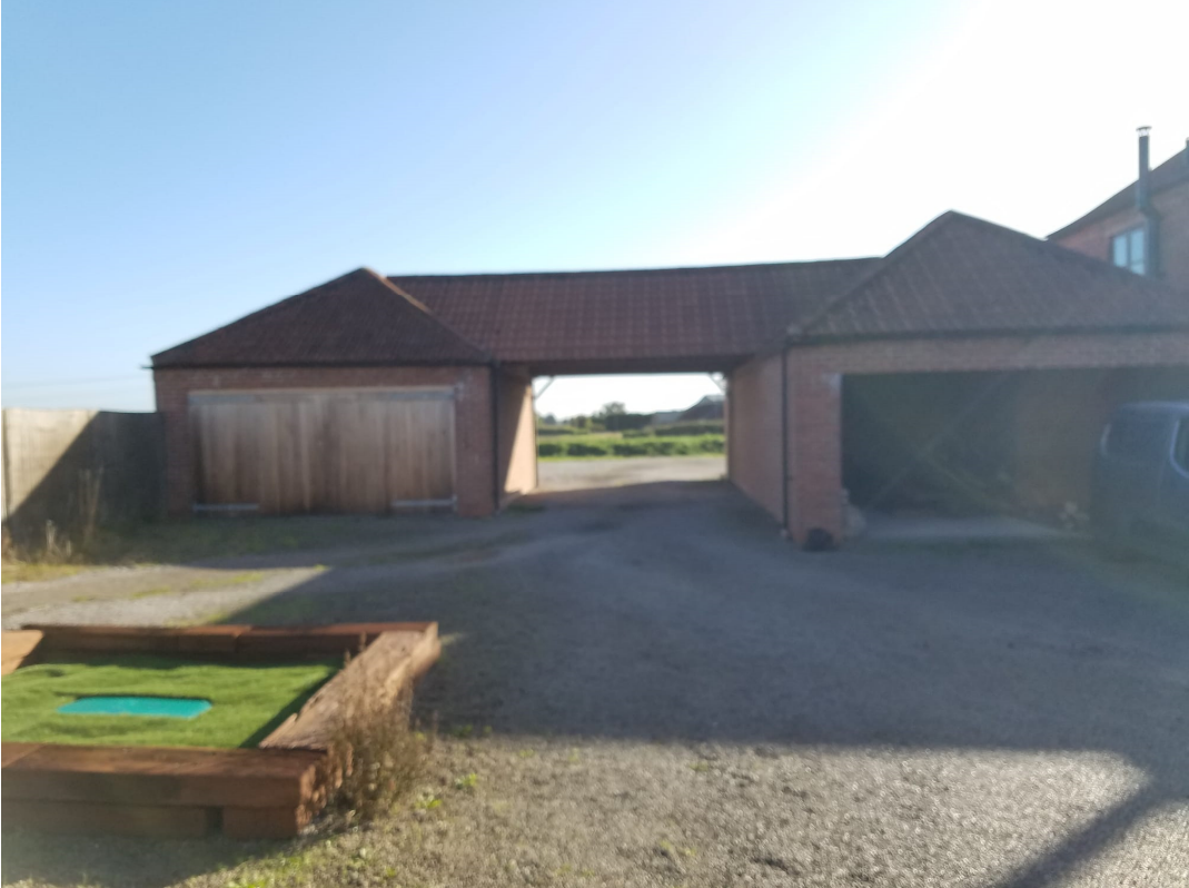
Photograph 1 Showing Existing Front Elevation to Garages 1 and 3 Prebendary Farm
