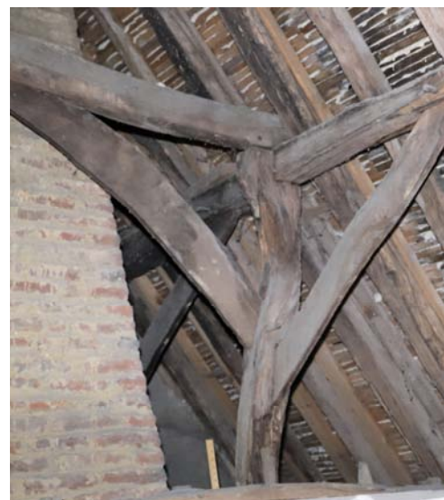
Fig 26: South queenpost on truss BB'
