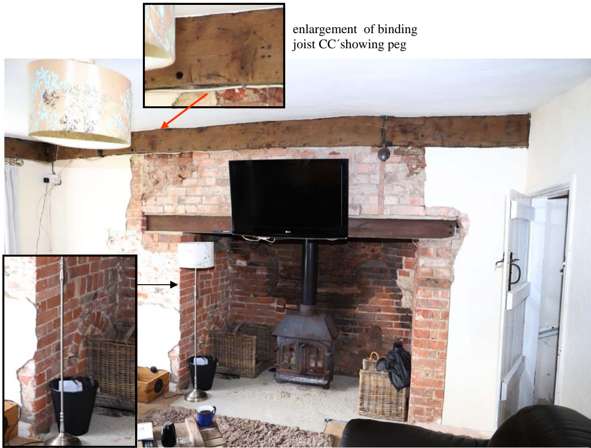
Fig 7: Hall fireplace with evidence of an oven to left and corbelling for the stairs to the right
