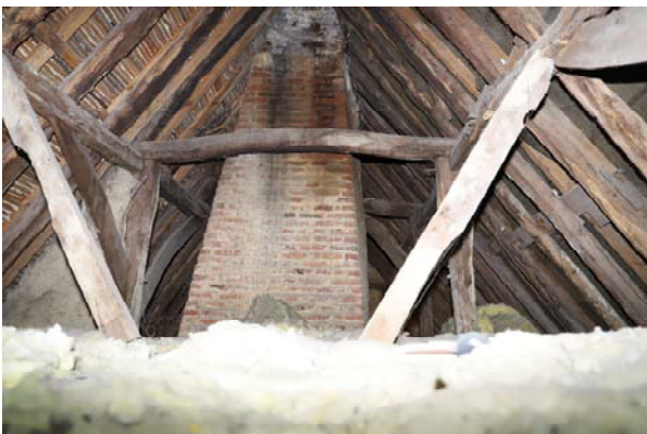
Fig 23: Truss CC' looking west
