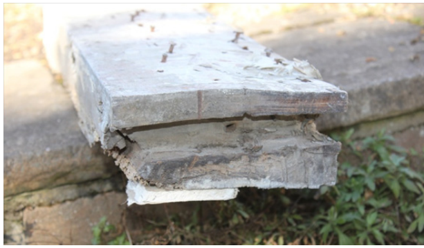
Fig 2: Top of stud grooved for wedge in Nayland, Suffolk (photo by Andrea Kirkham)
