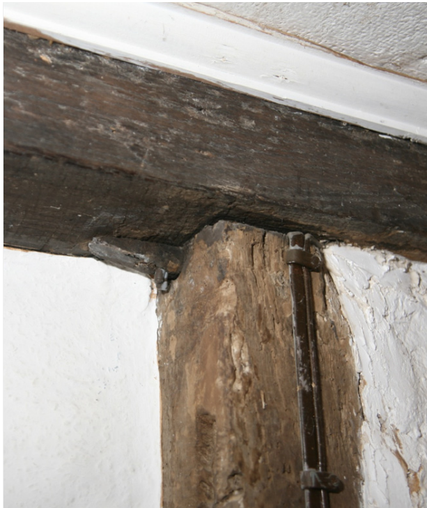
Fig 3: Wedged partition around chimney in early 17 th century lobby entrance in Stutton, Suffolk
