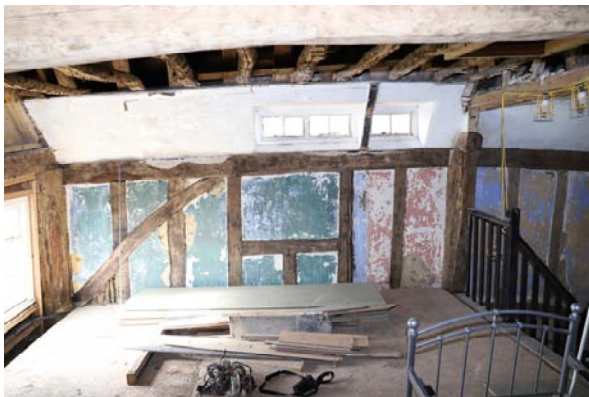
Fig 17: Rear wall of parlour chamber
