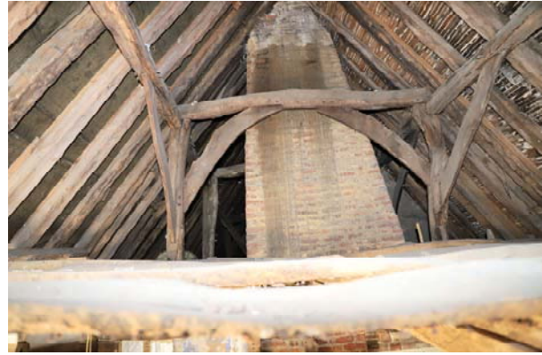
Fig 22: Truss BB' looking east
