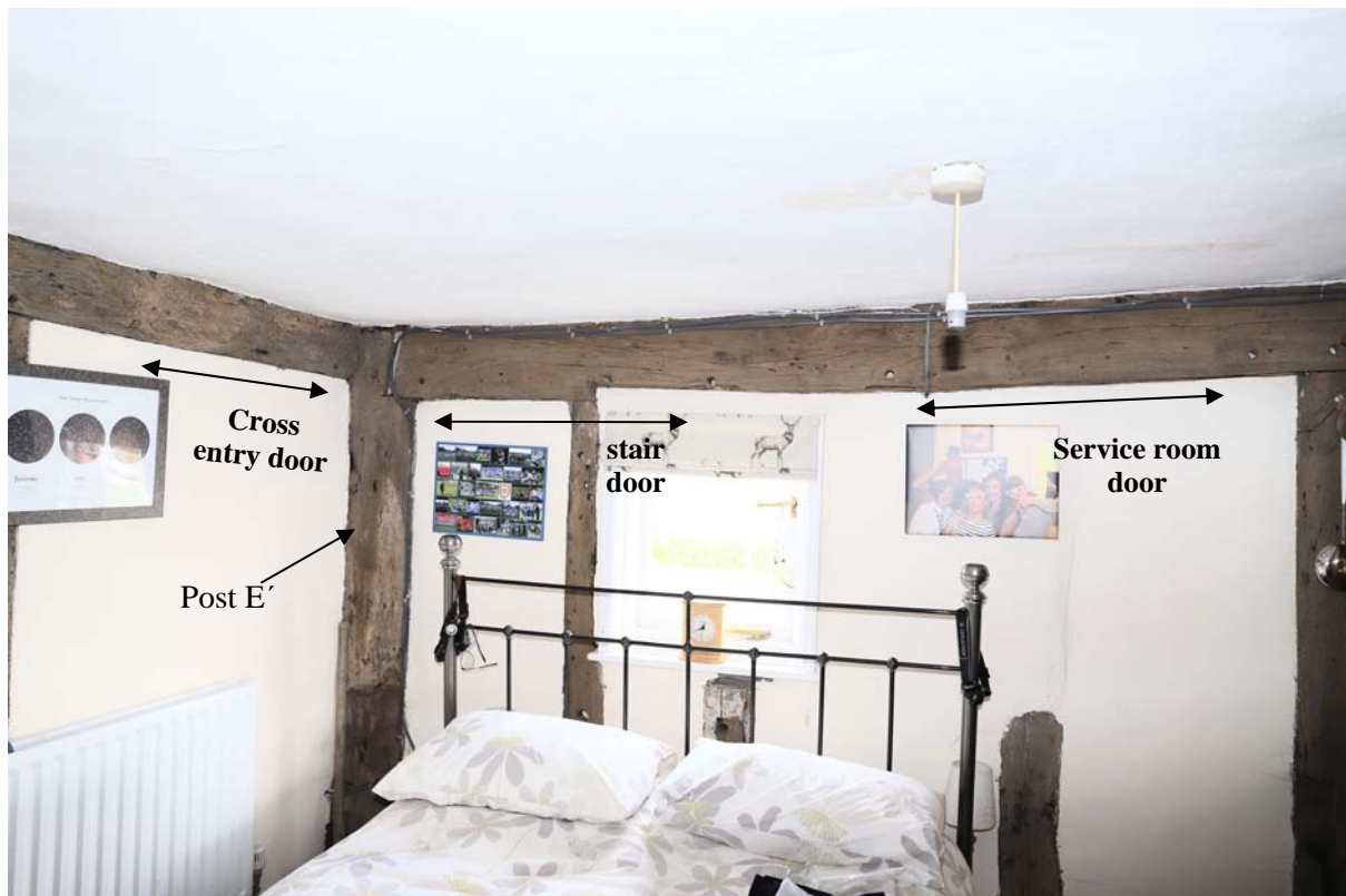
Fig 5: North-east corner of hall on ground floor (left the north cross entry door; right of principal post E' the doors to the stair & service end)
