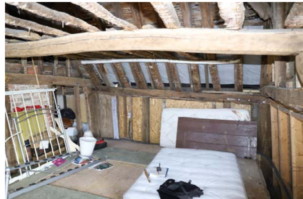
Fig 18: Front wall of parlour chamber
