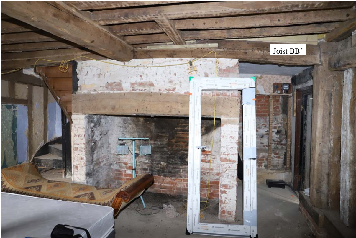
Fig 11: Parlour fireplace with immediately in front of it two cut common joists.
