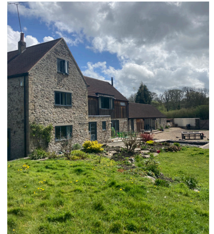
Fig 15: Rear of the property, facing W
