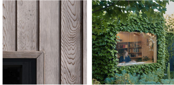
Untreated cedar cladding to match the existing building - the intention is to grow plants up the frontage of the extension to encourage a rich biodiversity and wildlife.
