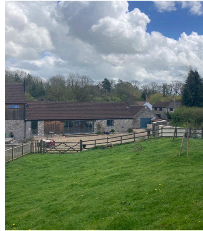
Fig 12 : Rear of the property facing SE
