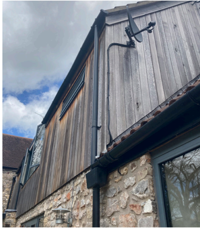
Fig 8 : West side of the property
