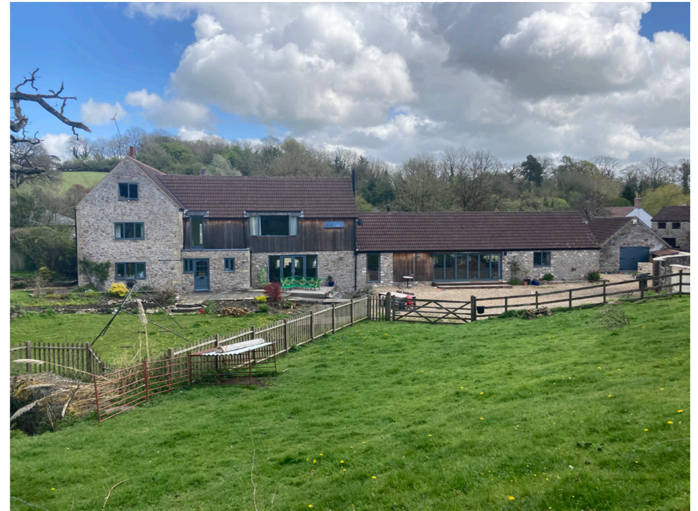
Fig 7: View of the west side of Vobster House - the gabion protected floodgate is shown in the foreground.
