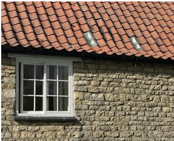
Existing glass tiles on the front elevation.
