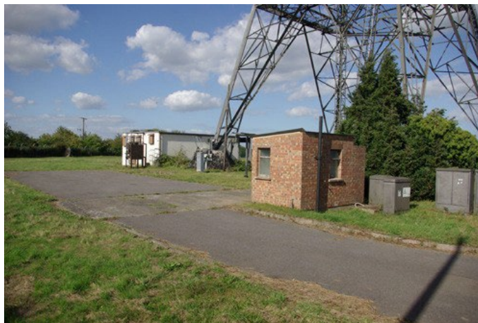
Figure 10 The toilet block to the south of the mast, looking north-west.
