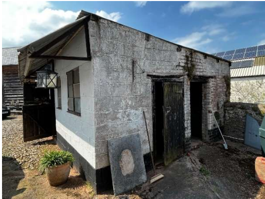
Plate 2. South-eastern elevation of the building
