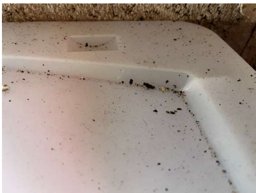
Plate 6. Bat droppings found within the central storage room
