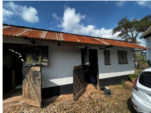
Plate 3. Southern elevation of the building
