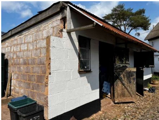
Plate 4. Western elevation of the building
