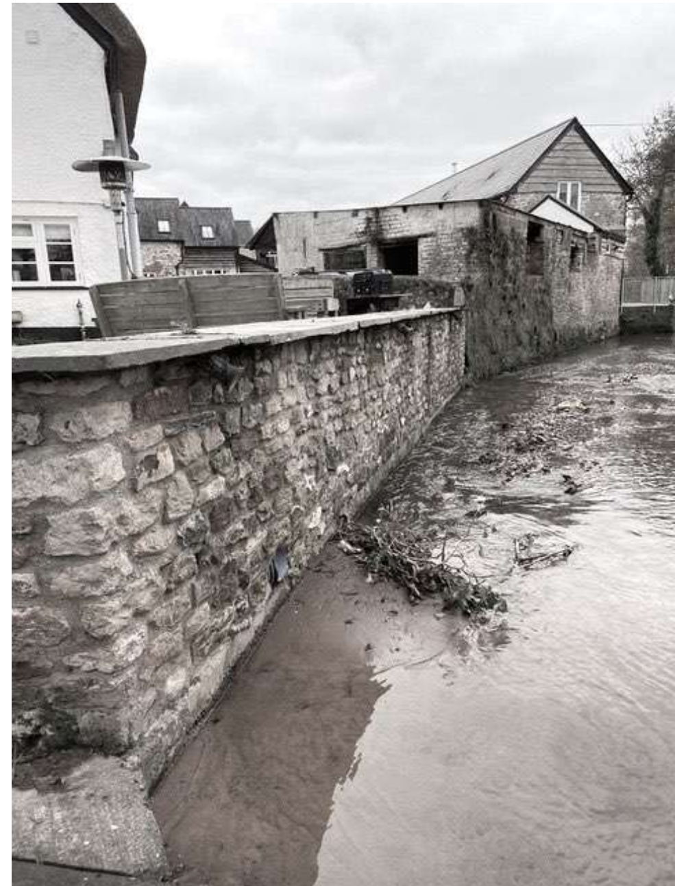
Fig 3: Existing stables looking South West along side the river Ken
