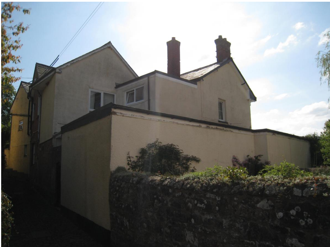
The north west corner of the existing apartment
