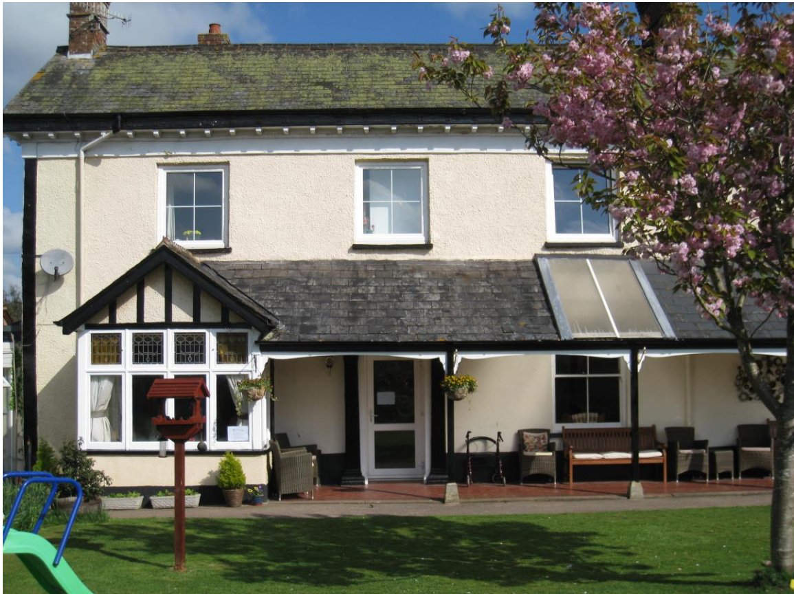
The existing residents' conservatory & veranda which are to be replaced
