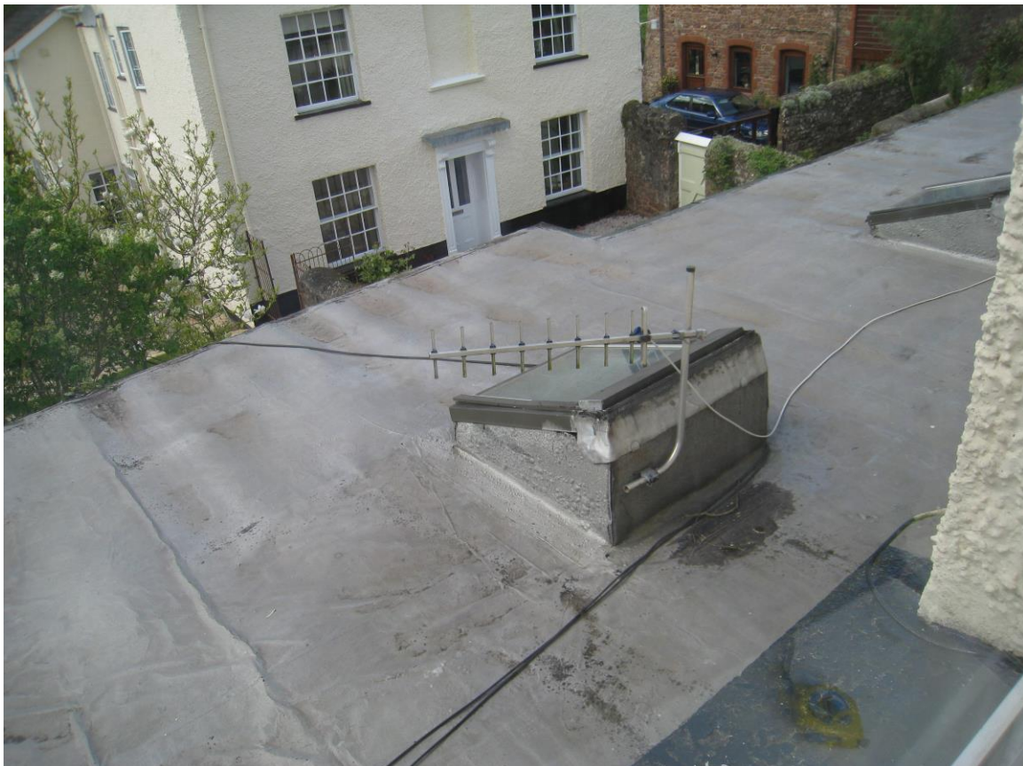
The existing apartment flat roof showing the unsightly roof lights
