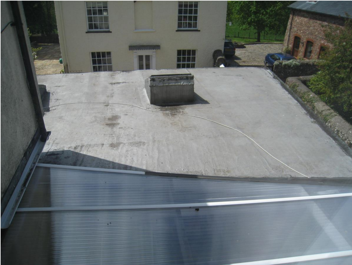
The existing apartment flat roof and roof over the kitchen courtyard
