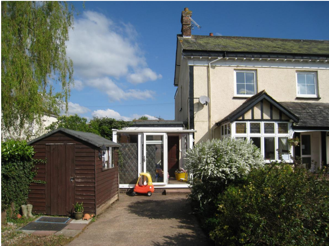
The existing concrete path over which the new extension is to be built
