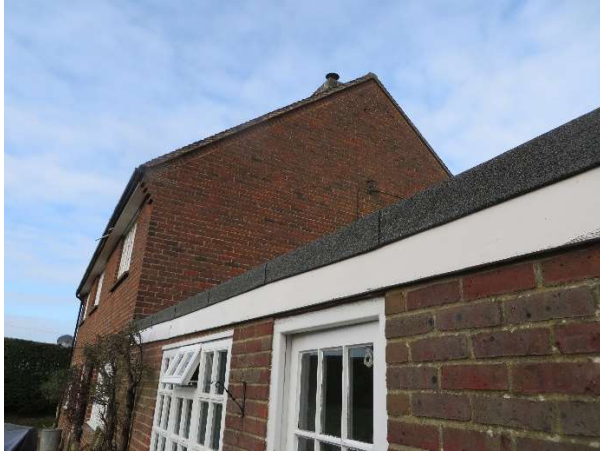
Showing flat roof of garage to be removed and the closed gable verge construction which will be covered over by the extension.
