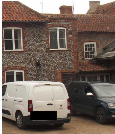
Extension linking rear building (left) to house service wing (right)
