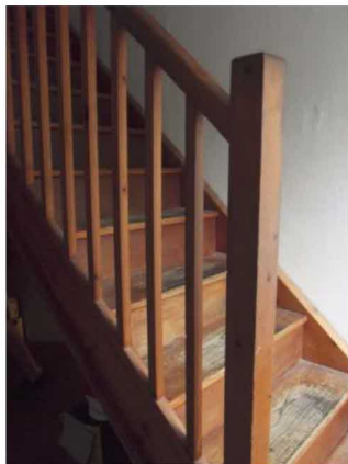
Stair in south extension
