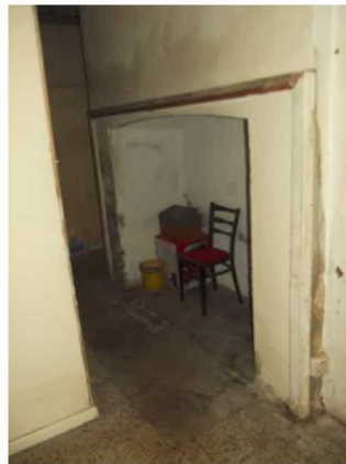
Fireplace in N section
