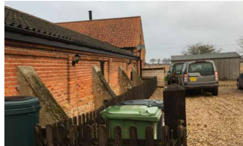
View N at Churchview Barn Access Drive/Gate
