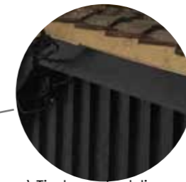
a) Timber cladding, eaves with wet verges
