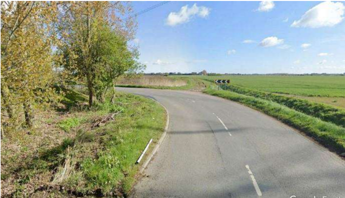
Figure 9. St Paul's Road South looking west at tight left-hand bend
