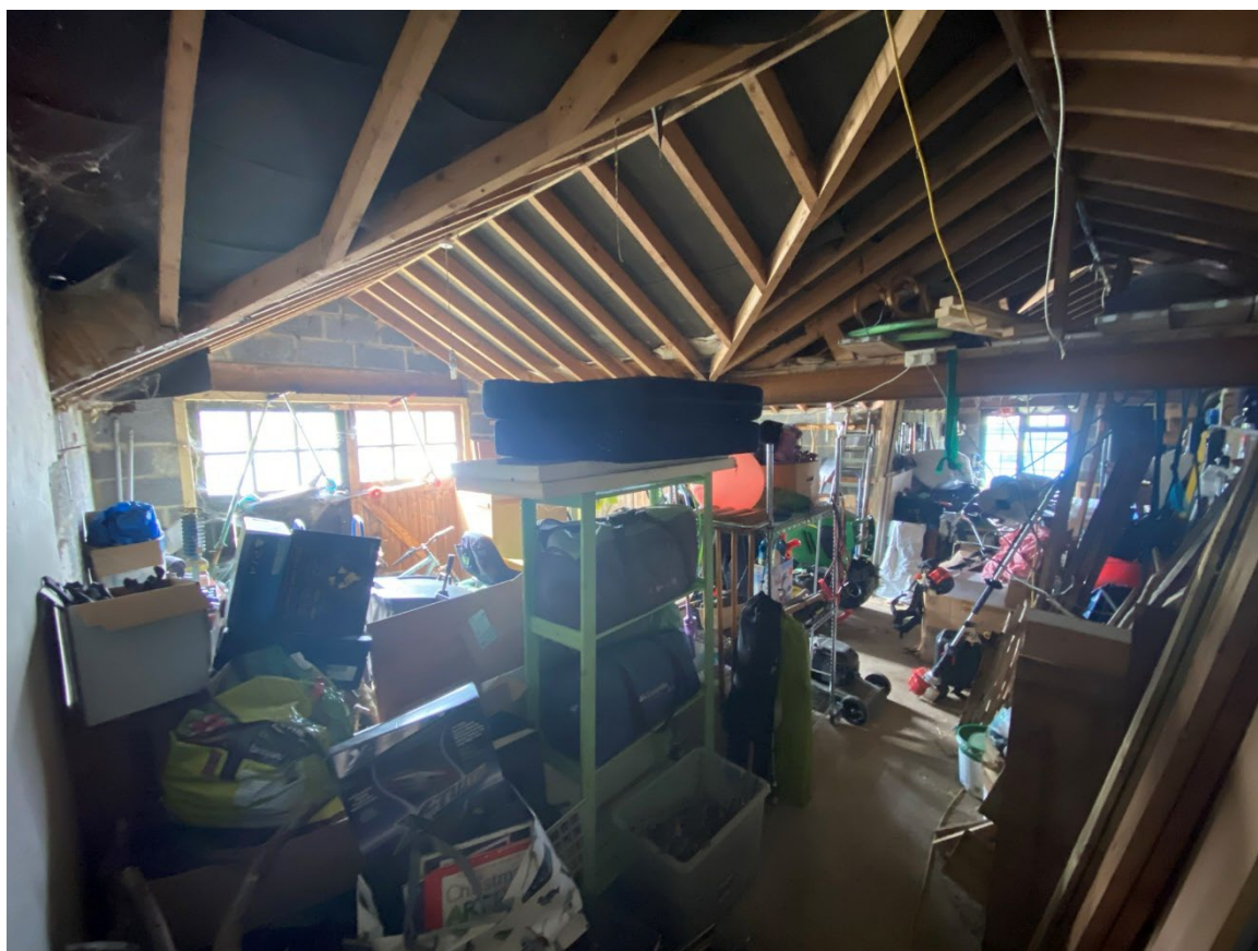
The existing garage / workshop
