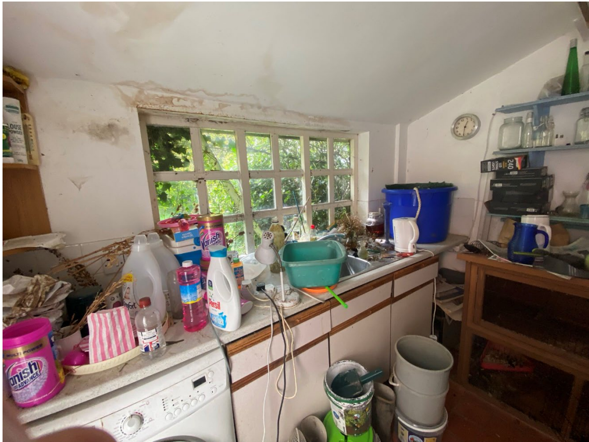
The existing utility room
