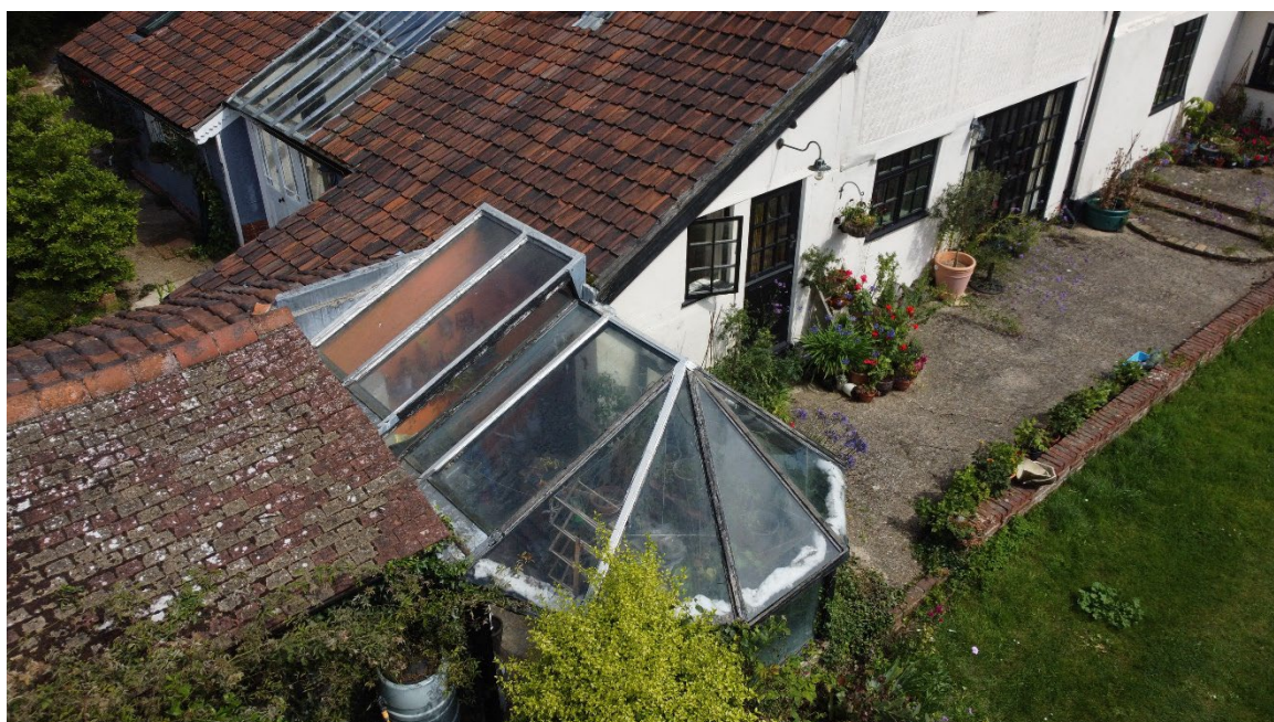
The existing conservatory
