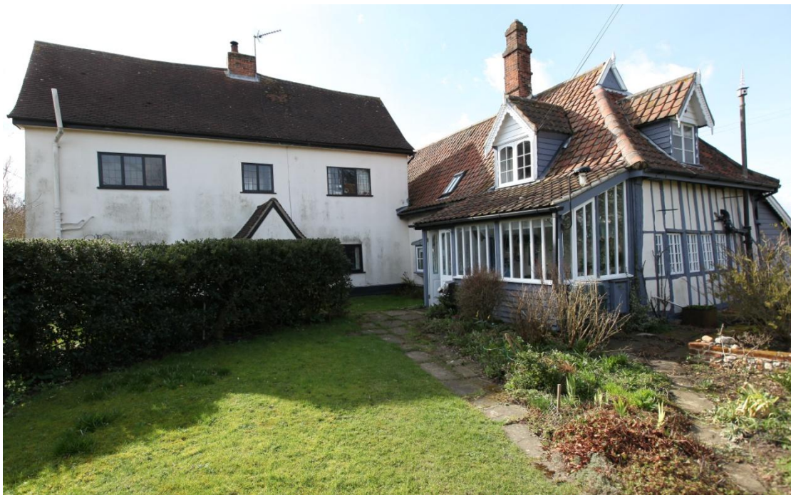
Illus. 2. The original north-eastern facade with the complete early-16 th century 1.5 storied house on the right and the two-storied 17 th century extension that probably formed a 'unit' house in front of its parlour on the left. No. 1 comprises the extension and the 16 th century ground-floor parlour. Note the dramatically reduced size of the chimney since 1964.
