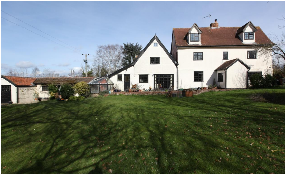
Illus. 4. The house from the site of the demolished farm buildings to the west with the formerly hipped parlour gable of the original house in the centre and the various single-storied extensions of the 1980s on the left. These extensions form part of no. 1 along with the original ground-floor parlour lit by French doors and the two-storied addition to the right. The first-floor room above the parlour belongs to no. 2.
