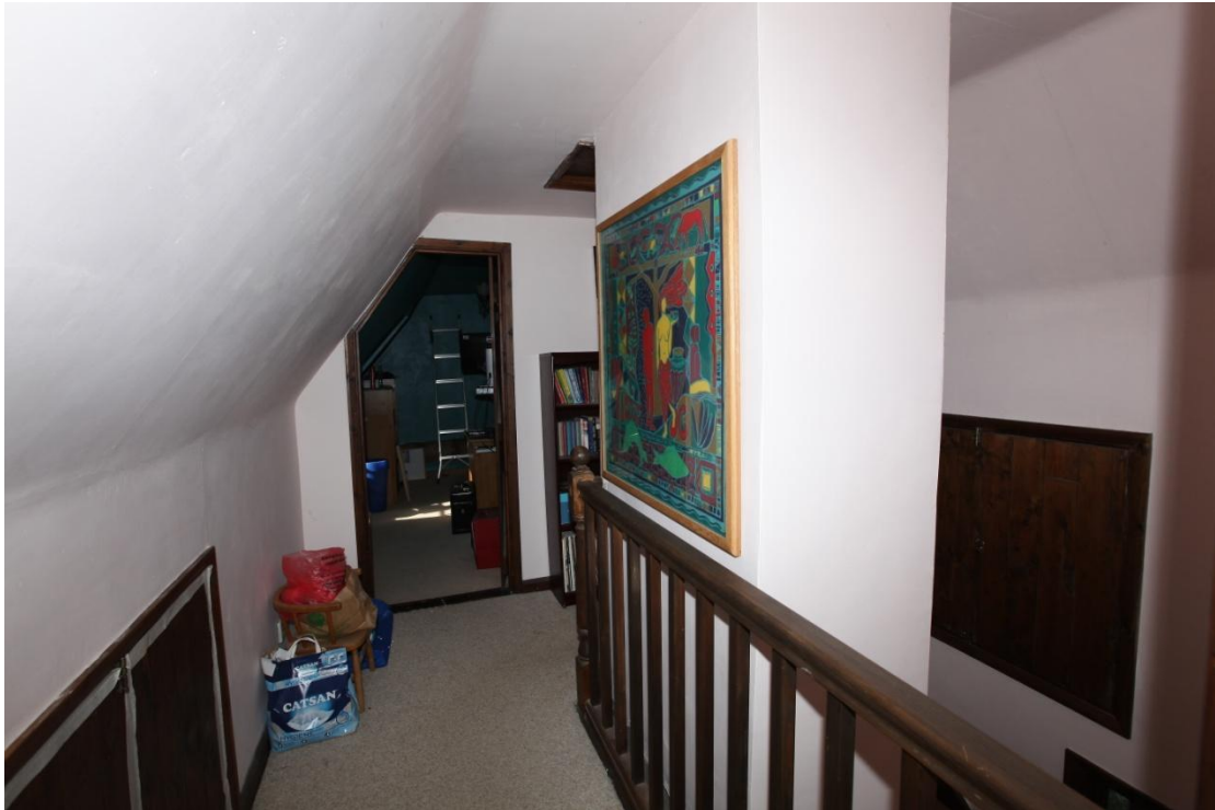
Illus. 21. The central stair landing of the attic storey, as seen from the south-east. The narrow Fletton-brick chimney, partitions and balustrade date only from the 1980s, as do the dormer windows to the south-west (left). The roof structure is hidden by plasterboard but a number of original rafters are visible above the ceiling and retain traces of soot-encrustation having been re-used from a medieval open hall.
