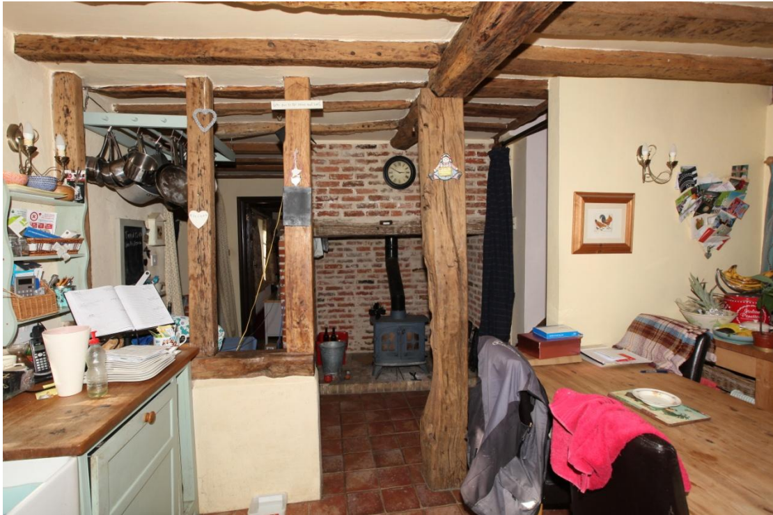
Illus. 15. The kitchen (3) from its south-eastern gable showing the re-used timbers of a partition that was probably inserted in the 1980s to frame the staircase on the right of the fireplace.
