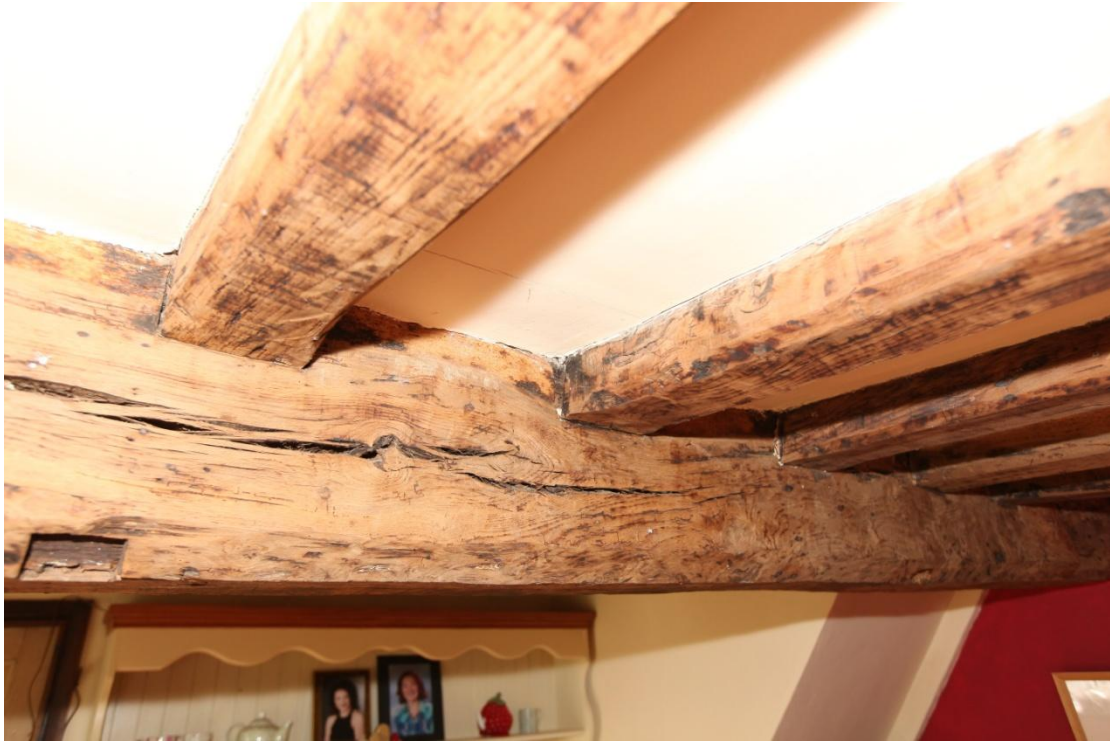
Illus. 7. A detail of the chamfered ceiling joists with small step-steps in the early-16 th century parlour (1). The timber has been cleaned by abrasion.
