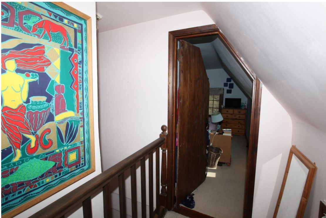
Illus. 22. The attic stair landing looking towards the south-eastern gable showing the late-20 th century balustrade and plasterboard partitions. This level of the house was previously lit by dormer windows in the north-eastern facade and has been altered almost beyond recognition.
