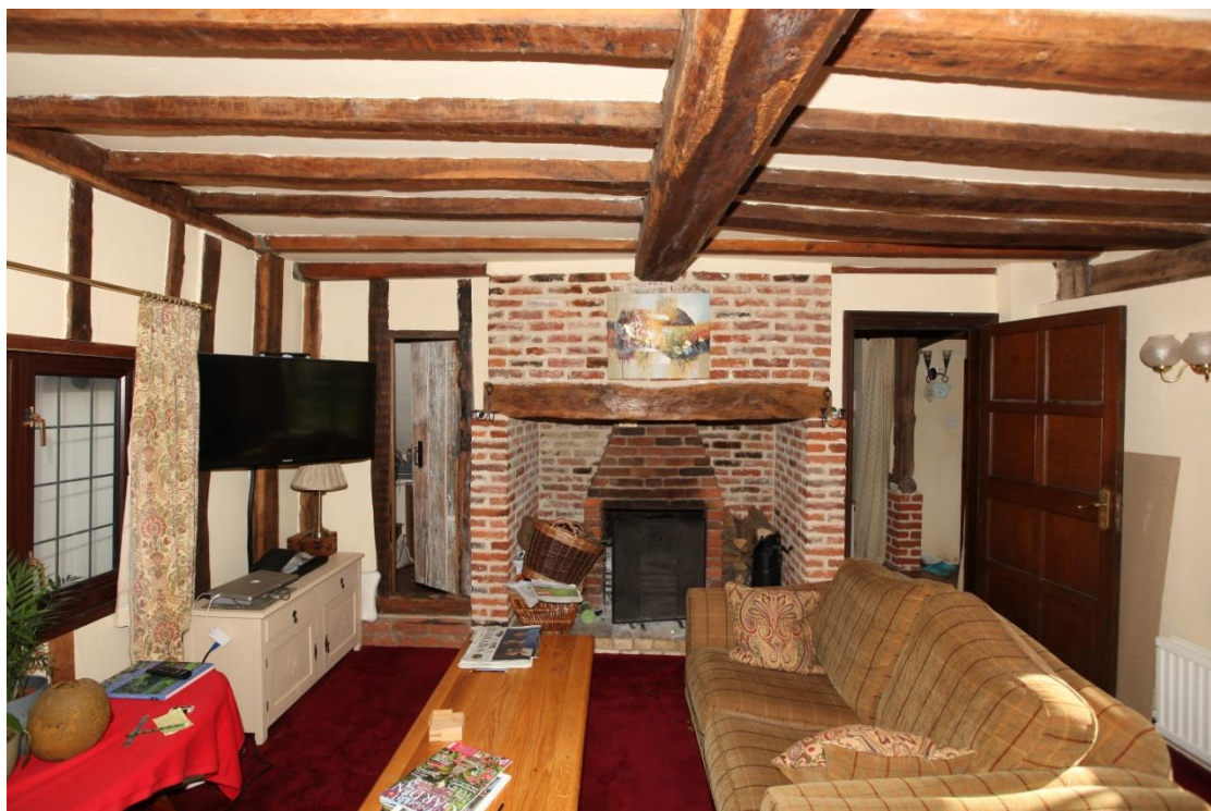
Illus. 10. The fireplace to the south-east of the sitting room (2), with lobbies on each side that open into the original porch on the left and its modern counterpart on the right. The fireplace consists of re-used bricks, some of which are soot-encrusted, and appears to date only from the late-20 th century. Curiously the tall-sectioned ceiling joists to the left of the room are tenoned to the mid-rail while their counterparts to the right are flat-sectioned in the earlier tradition and lodged on the mid-rail.
