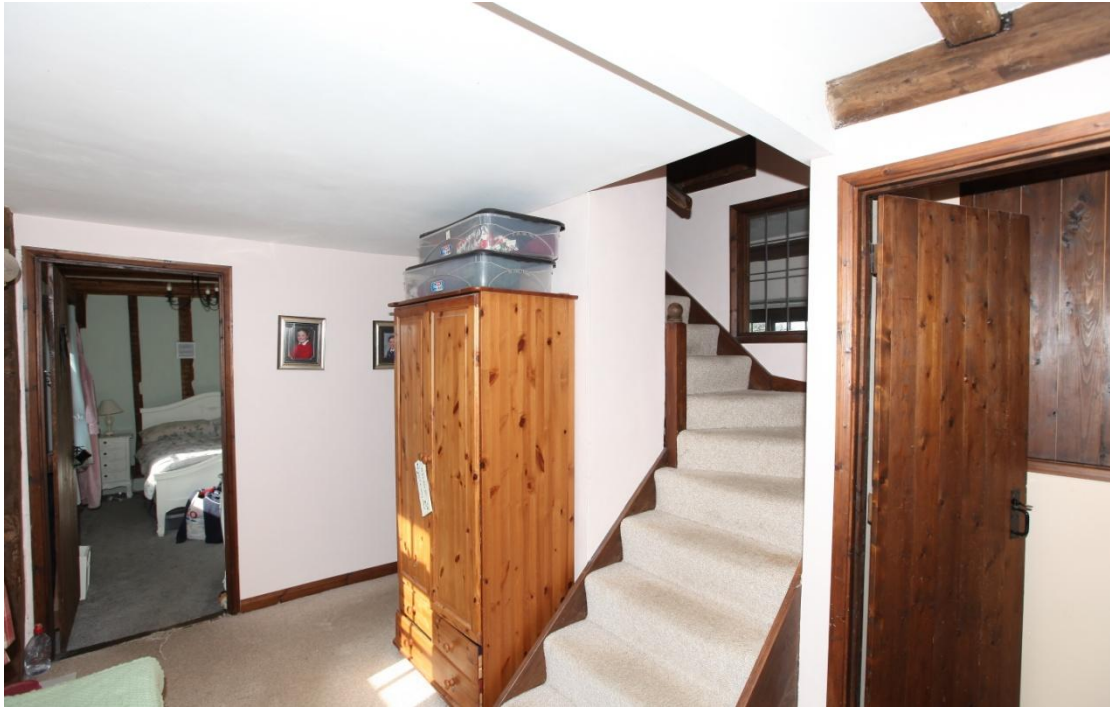
Illus. 19. The stair landing on the first floor as seen from the south-east with the narrow, rebuilt chimney of rendered Fletton brick in the centre. Like the chimney the internal partitions and doors at this level date almost entirely from the extensive refurbishment of the 1980s. The large original chimney in figure 7 would have contained 17 th century fireplaces heating the bedrooms rooms on each side.
