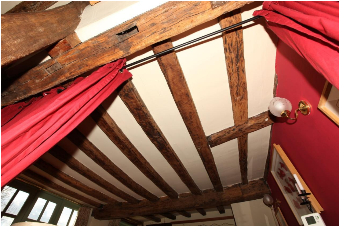
Illus. 8. The early-16 th century parlour ceiling (1) from the sitting room in its front extension (2). Empty mortices for the missing studs of the original front wall are visible in the mid-rail above with no gaps for windows. The stair in the blocked trap would have risen from the foot of the original doorway to the hall on the extreme right in a standard late-medieval arrangement.
