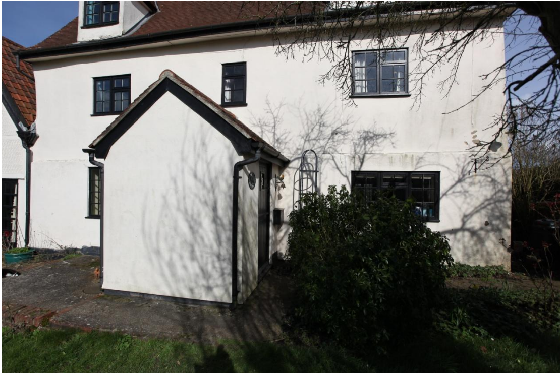
Illus. 5. The orientation of the house was altered as part of a major refurbishment in the 1980s which included the insertion of new dormer windows in the original rear (south-western) elevation and the addition of a new porch with a side-entrance facing the road. The ground and first-floor windows were renewed at the same time and the lower storey rebuilt in cement-rendered brick or block-work.
