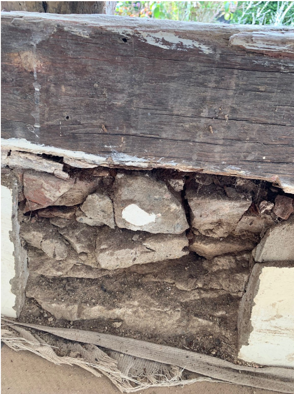
Sitting Room – West Elevation (note concrete & rubble infill)
