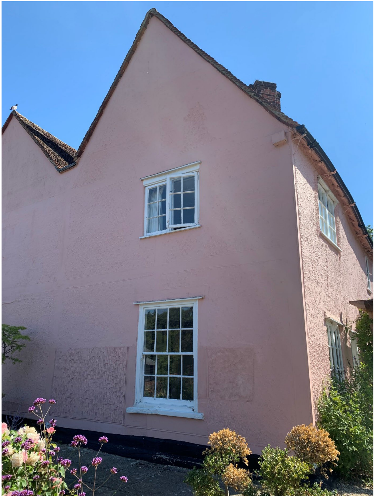
Master Bedroom, West Elevation – first floor bedroom window
