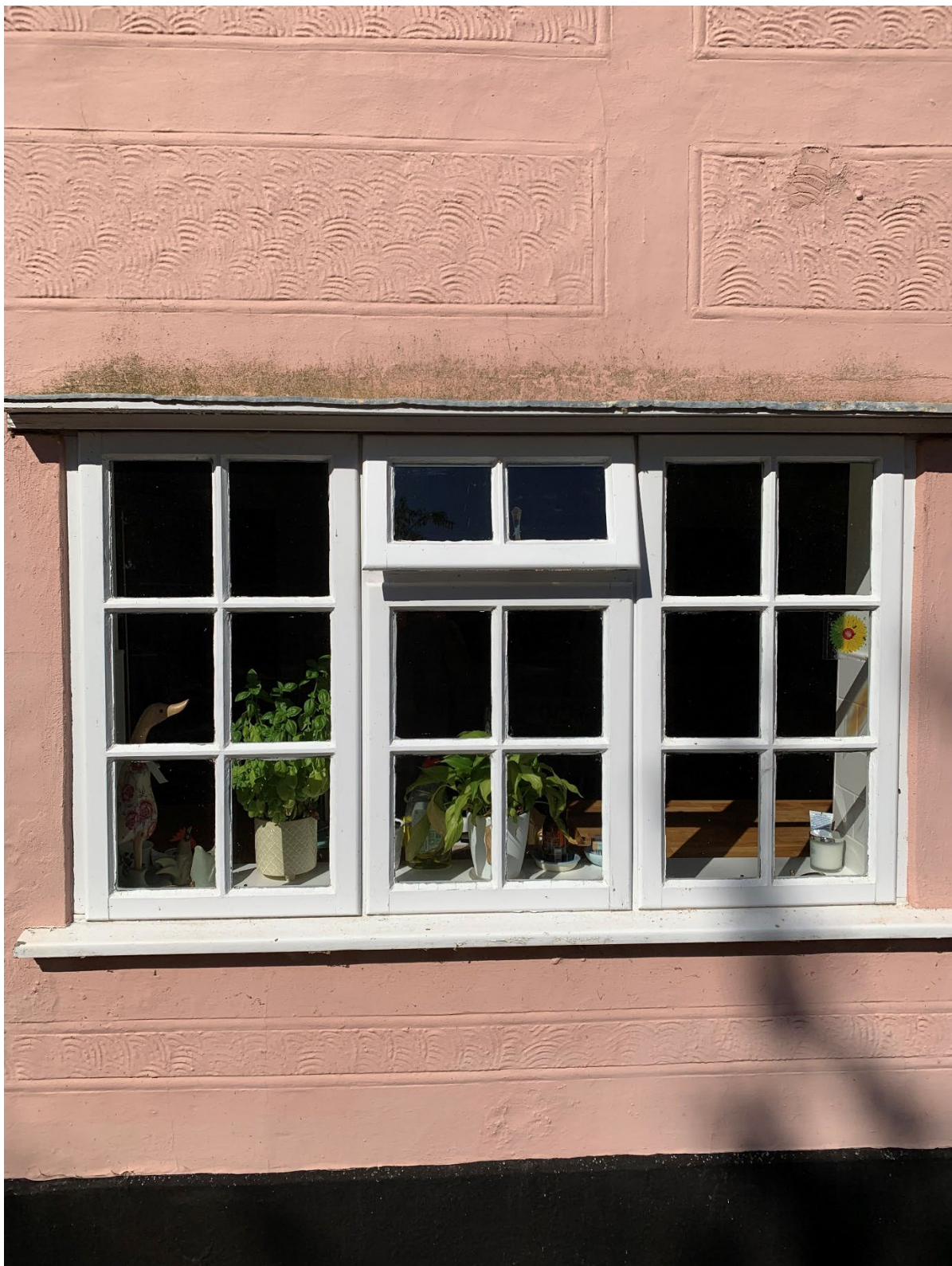
Kitchen, East Elevation – ground floor window
