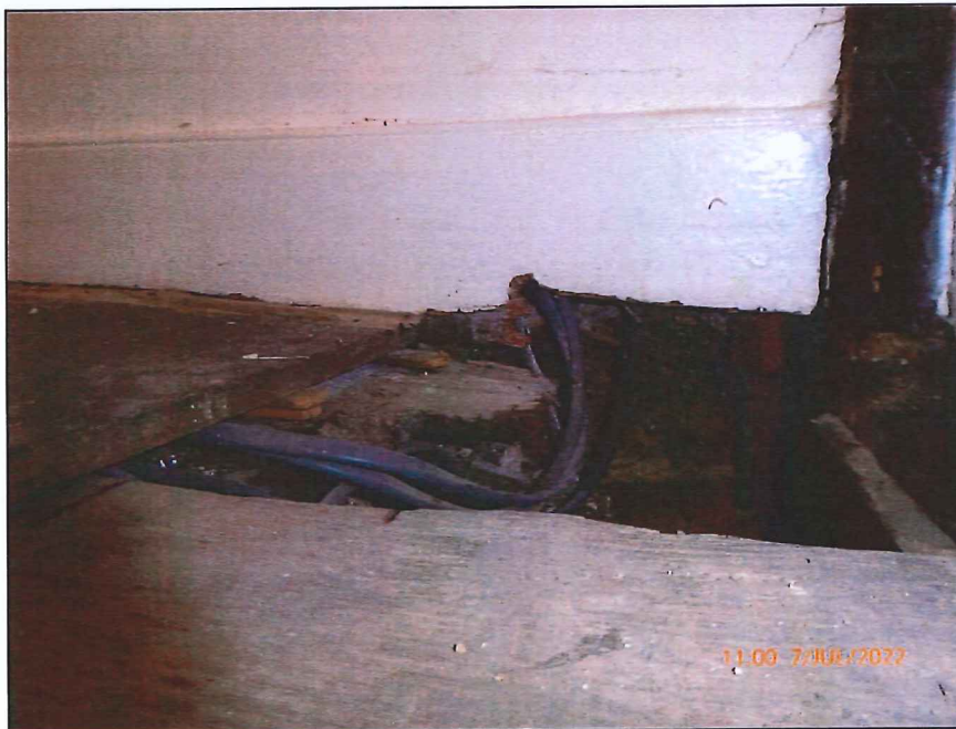
Photograph 14 – Corner Post at 1 st Floor
