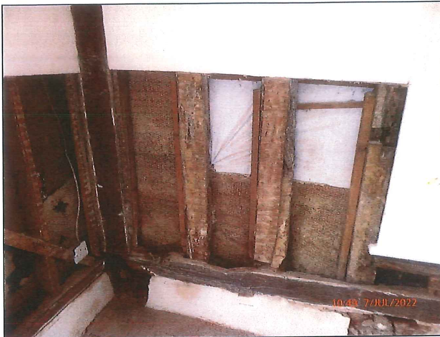
Photograph 7 – Corner/Side Wall Soleplate
