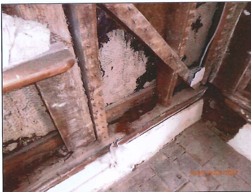
Photograph 10 – Corner Rear Wall
