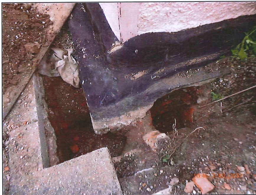
Photograph 18 – External Trial Hole
