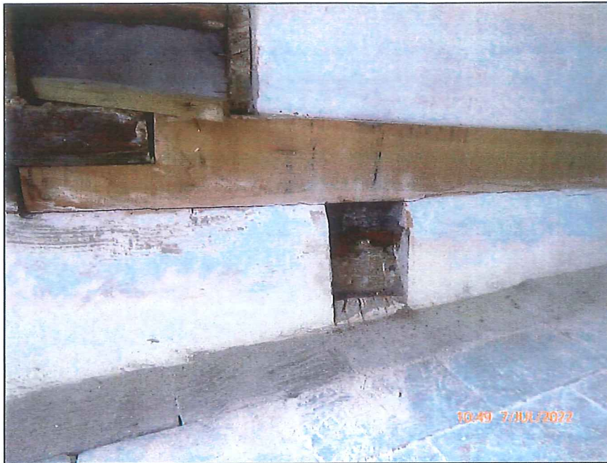
Photograph 15 – Side Wall Replacement Soleplate
