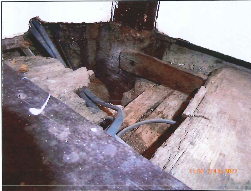
Photograph 13 – Corner Post at 1 st Floor
