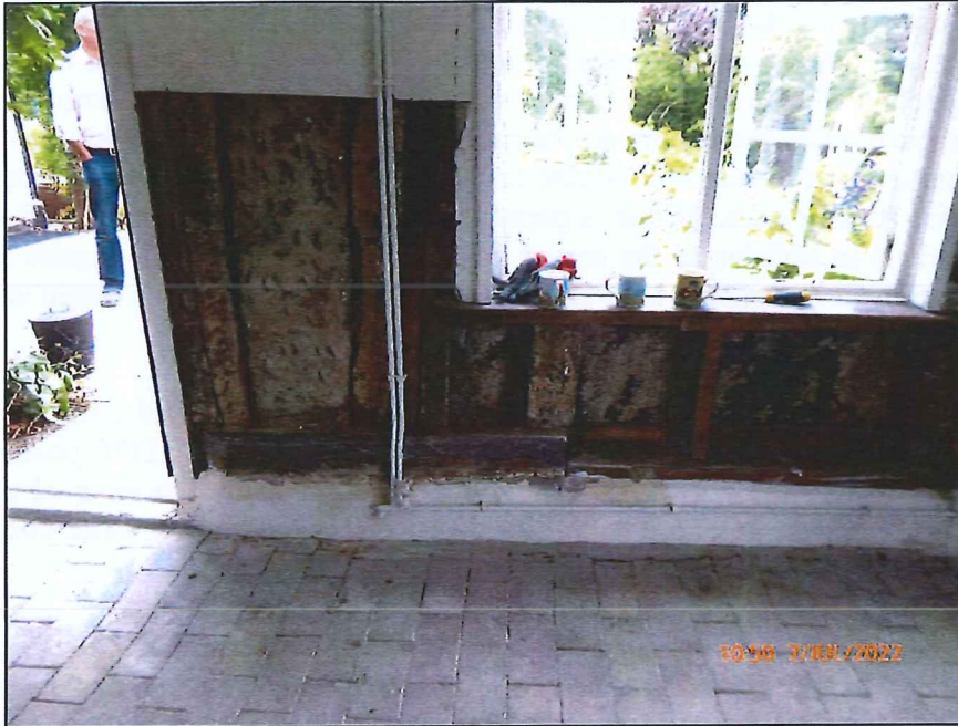
Photograph 1 – Living Room, Rear
