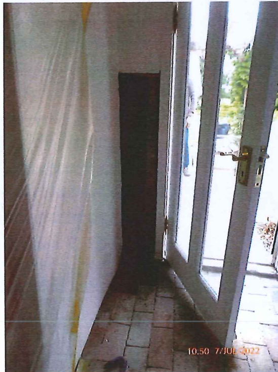
Photograph 6 – Living Room, To Left Hand Side of Door
