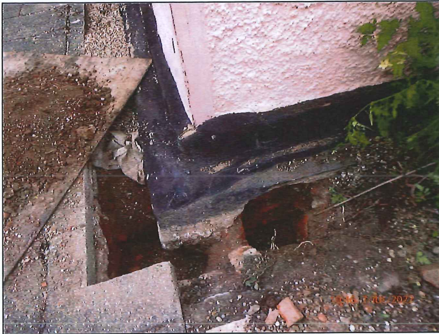
Photograph 17 – External Trial Hole
