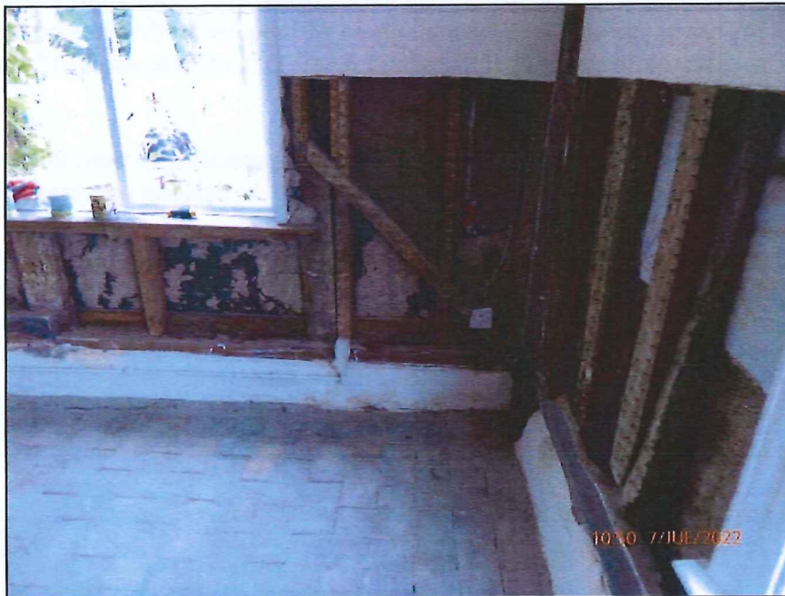
Photograph 2 – Living Room, Rear
