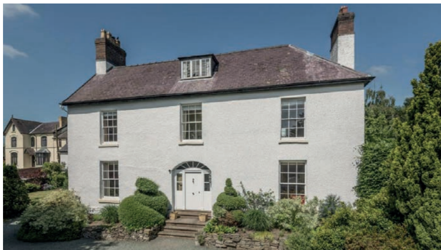
Another example of the off-white render and the grey slate working well together to uplift the dwelling and giving it feeling of grandeur.
