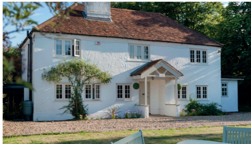
This is a great example of the pitched canopy front entrance which will create a sense of arrival and increase its presence to the street edge.
