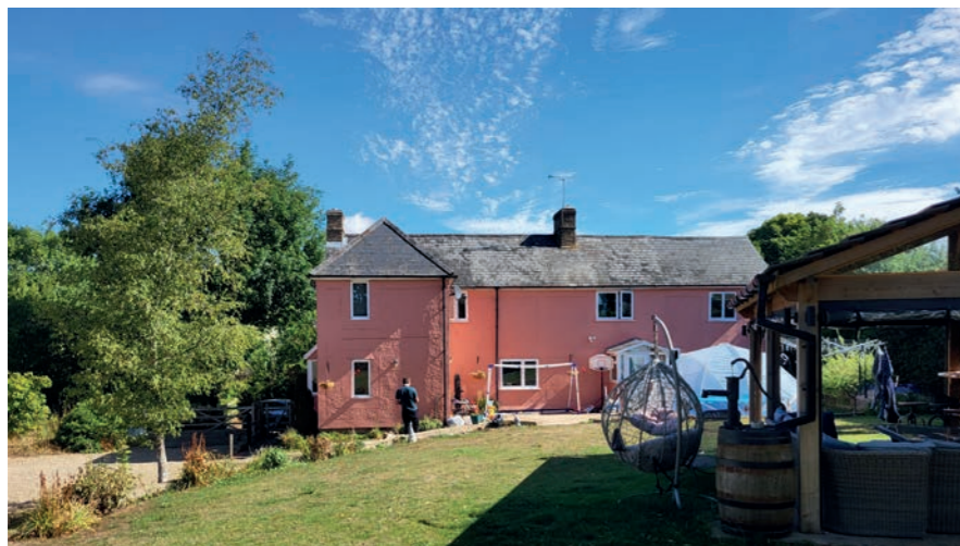
Existing Rear Elevation (Taken from the Rear Garden)
