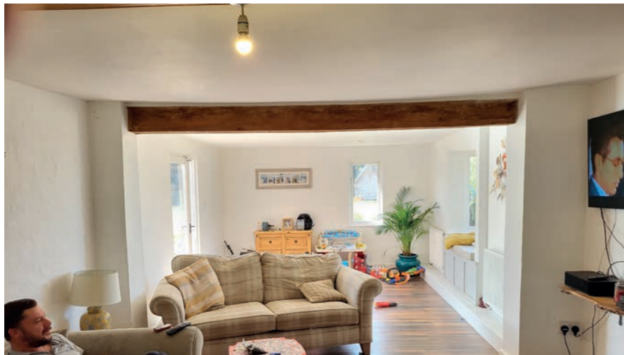
Beam visible internally showing where the new extension has been added
