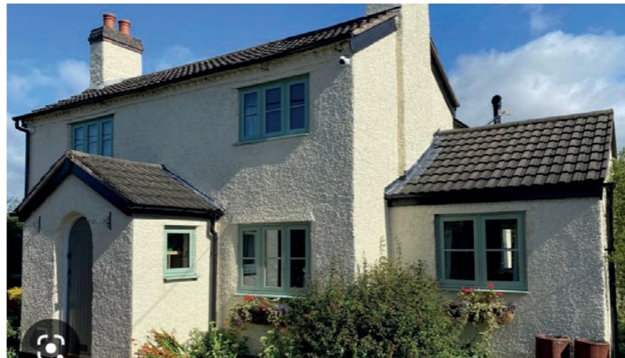
The teal window frames and off white render give the farm house a modern finish while retaining its character.
