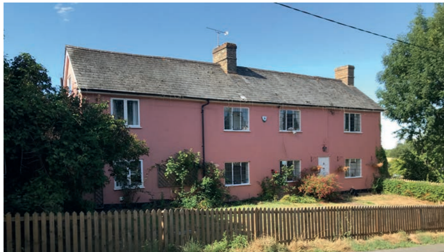
Existing Front Elevation (Taken from Hickford Hill)
