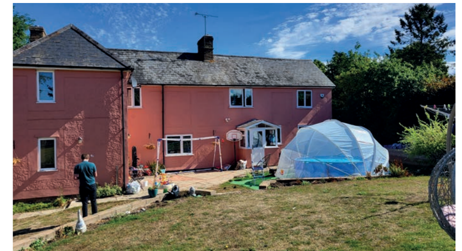
Rear elevation showing overgrown vegetation at the Eastern boundary.
