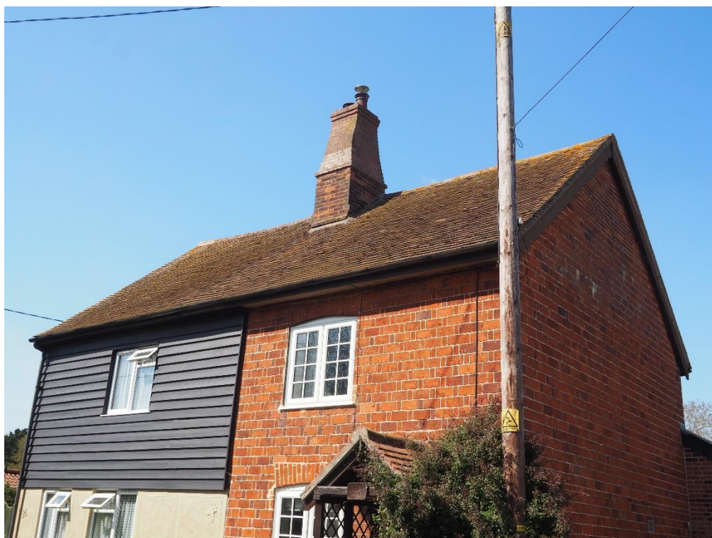
Figure 2: From Hicks Lane looking north-west towards 35 and 36 Hicks Lane.
