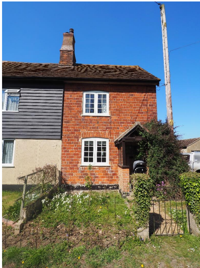
Figure 1: From Hicks Lane looking north towards 35 Hicks Lane.
