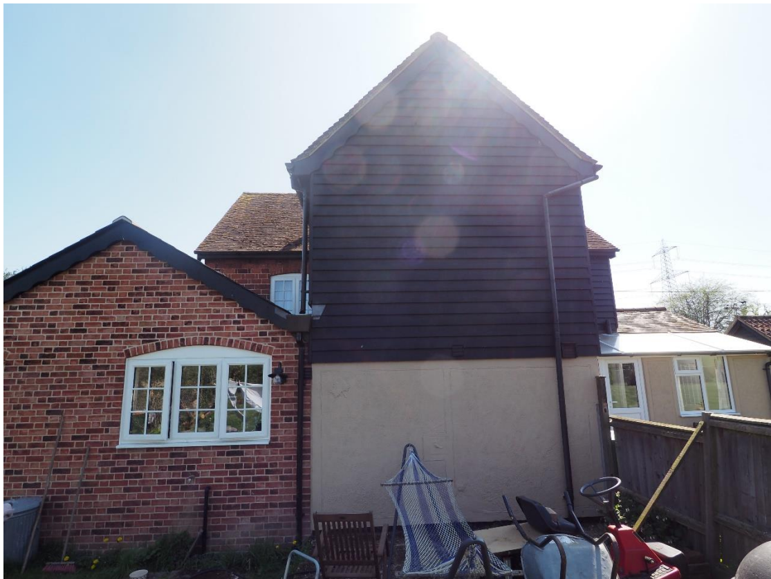
Figure 3: From rear garden looking south towards 35 and 36 Hicks Lane.
