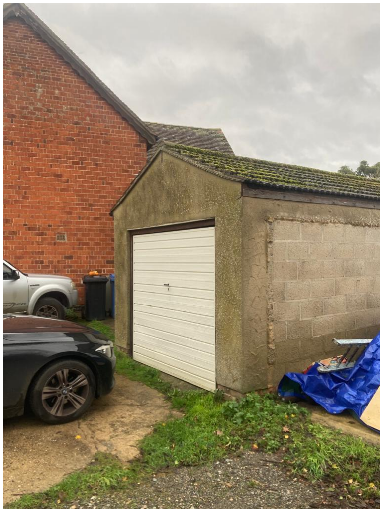
Figure 4: From driveway looking north-west towards existing garage (35 Hicks lane).
