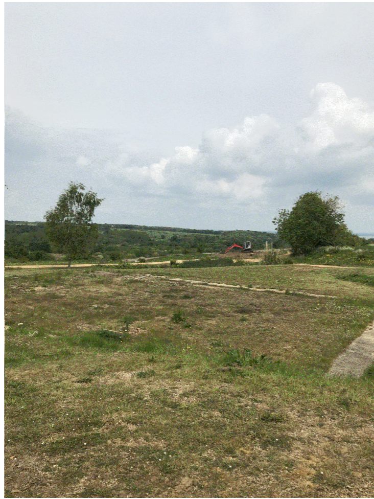
B - EXPOSED FOUNDATIONS TO HISTORIC BARN
