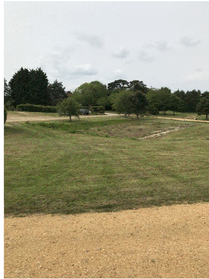
C - EXPOSED FOUNDATIONS TO HISTORIC BARN
