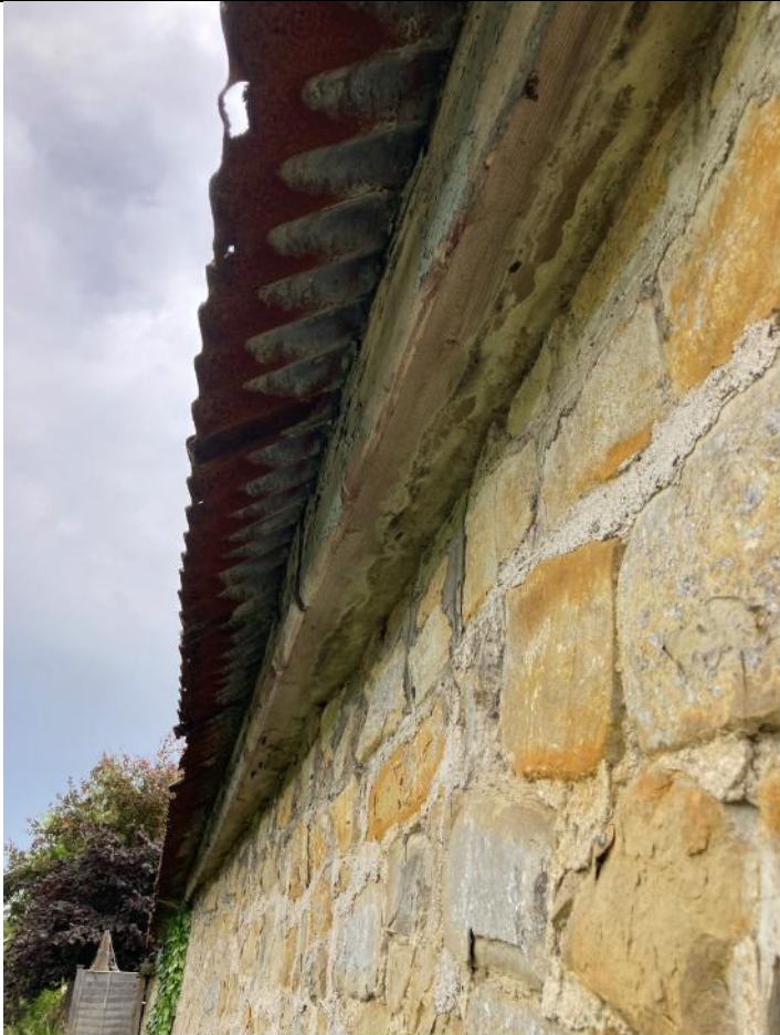
Photo 3: Looking east along the northern fascia.
