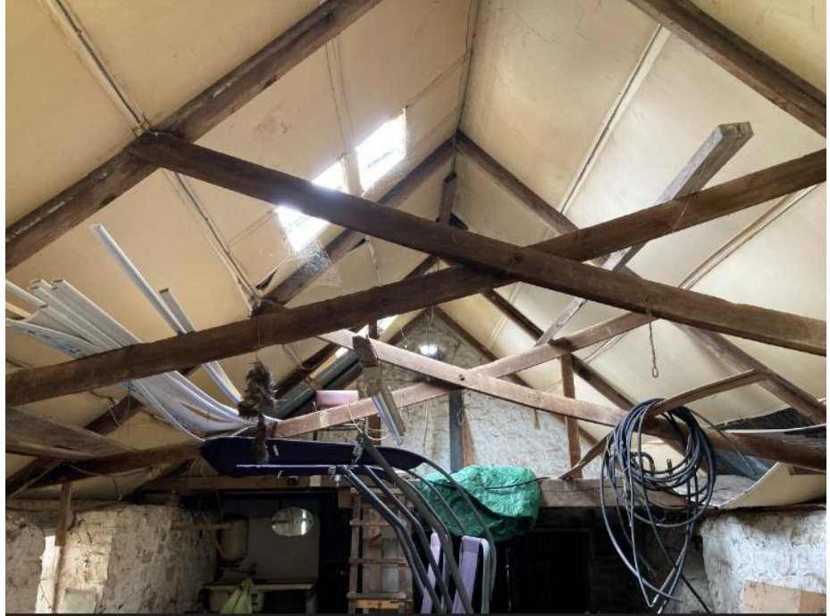
Photo 7: Looking west within the main building showing the internal roof structure.
