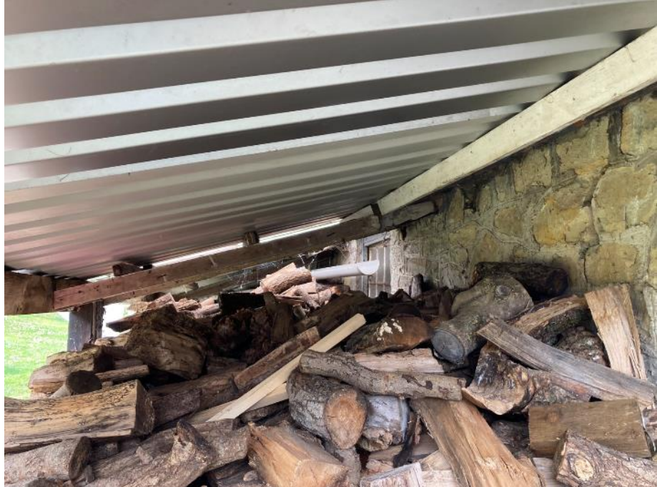
Photo 9: Showing the internal environment within the lean-to extension.
