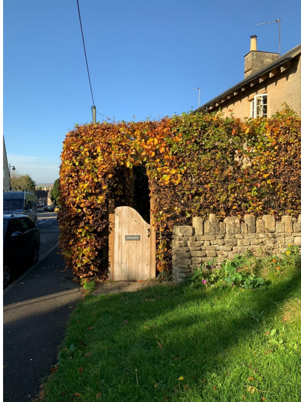
'Townsend' from the east showing gate to be removed and infilled (NB, the stone wall is a neighbouring property)
