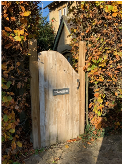
Modern pedestrian access gate to be removed
