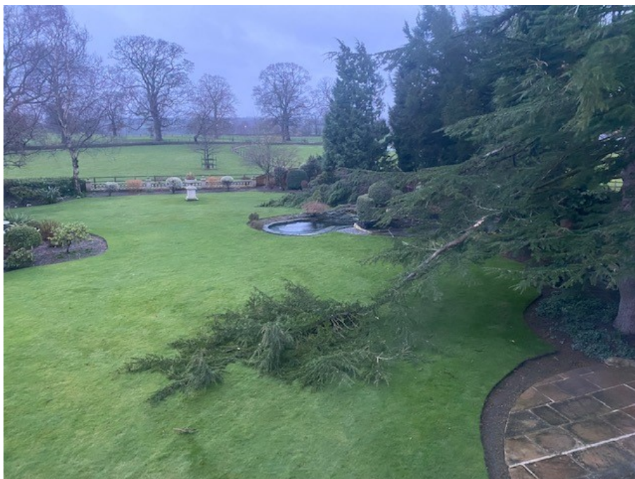
Photo A1.6 : View across the open land to the south and west of the estate wall at Bretton Lodge, showing tree damage caused by Storms Dudley and Eunice, February 2022.
