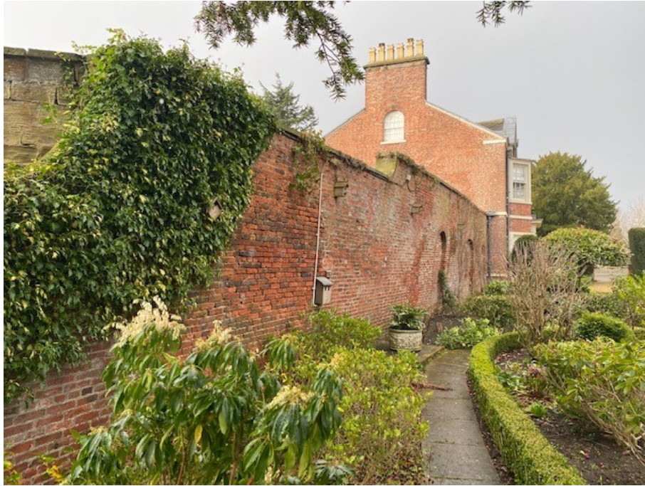
Photo A1.1 : The wall as viewed from the north-east.
