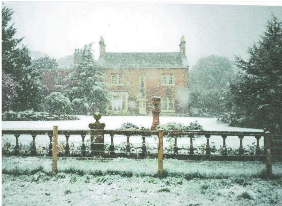
Photo A1.3 : Photo of Bretton Lodge taken in Easter 1998, showing the Atlas Cedar to the left hand side of the property. The estimated height of the tree at the time was 8m.
