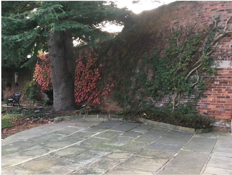
Photo A1.9 : The estate wall runs to the western side of the tree, and is of clay brickwork to its eastern face. NB also sandstone flagged patio area to the north of the tree.
