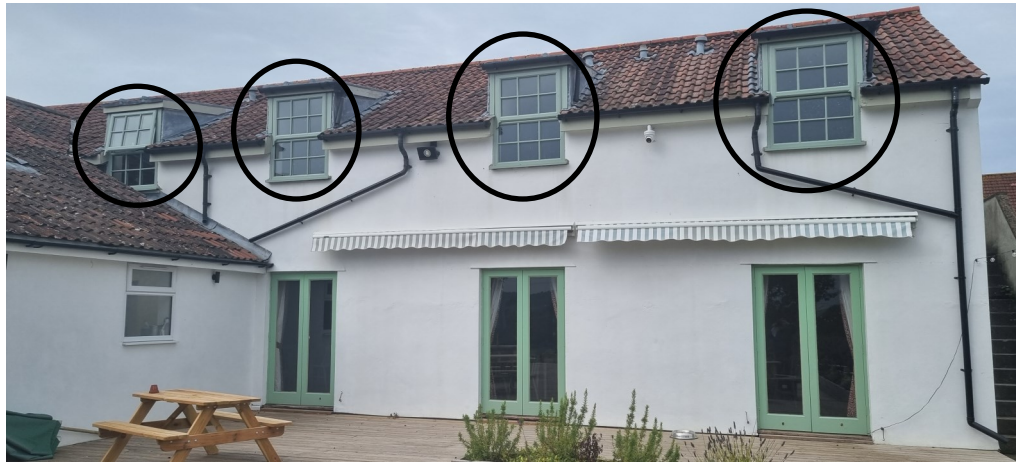
Photos 3-6: The 8 No. uPVC windows that were installed in June 2022 and are the subject of the replaced regularisation planning and listed building consent application are identified above. It is proposed to replace uPVC windows on an agreed, phased basis.
