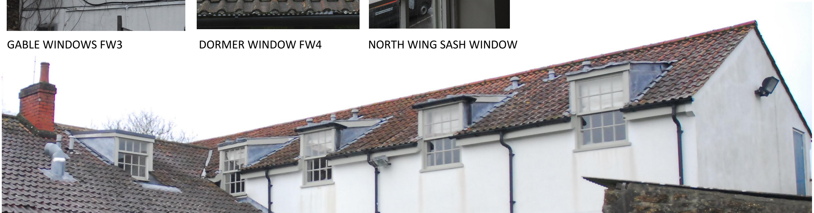
DORMER WINDOW FW4 AND NORTH WING REAR WINDOWS FW5, 6, 7 & 8
