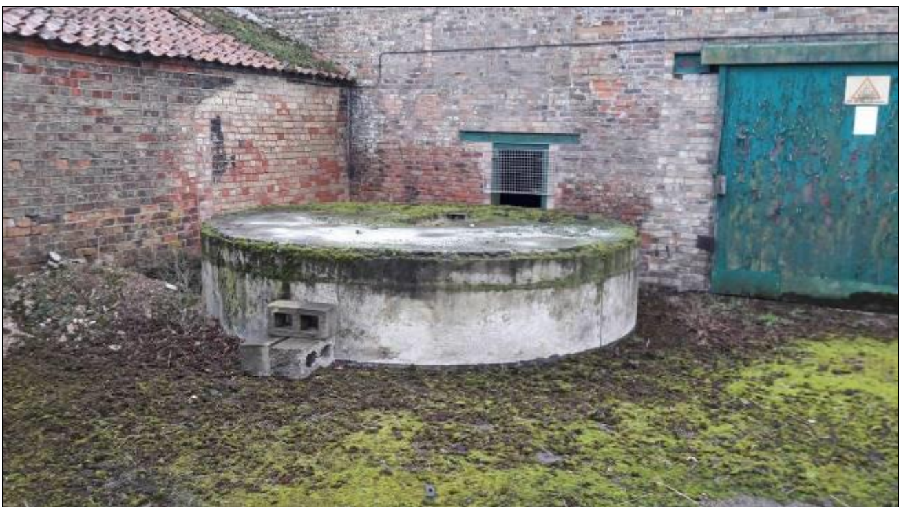
Fig 5 - concrete plinth of the former corn-feed silo
