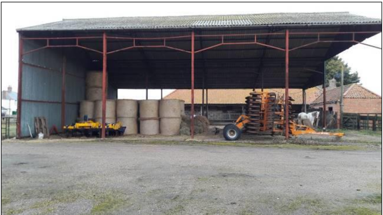
Fig 7 - view to the north of the former dutch barn, showing CBA-panels
