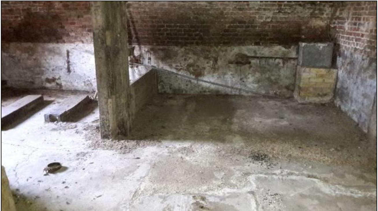
Fig 6 - interior of the barn showing the solid concrete floor
