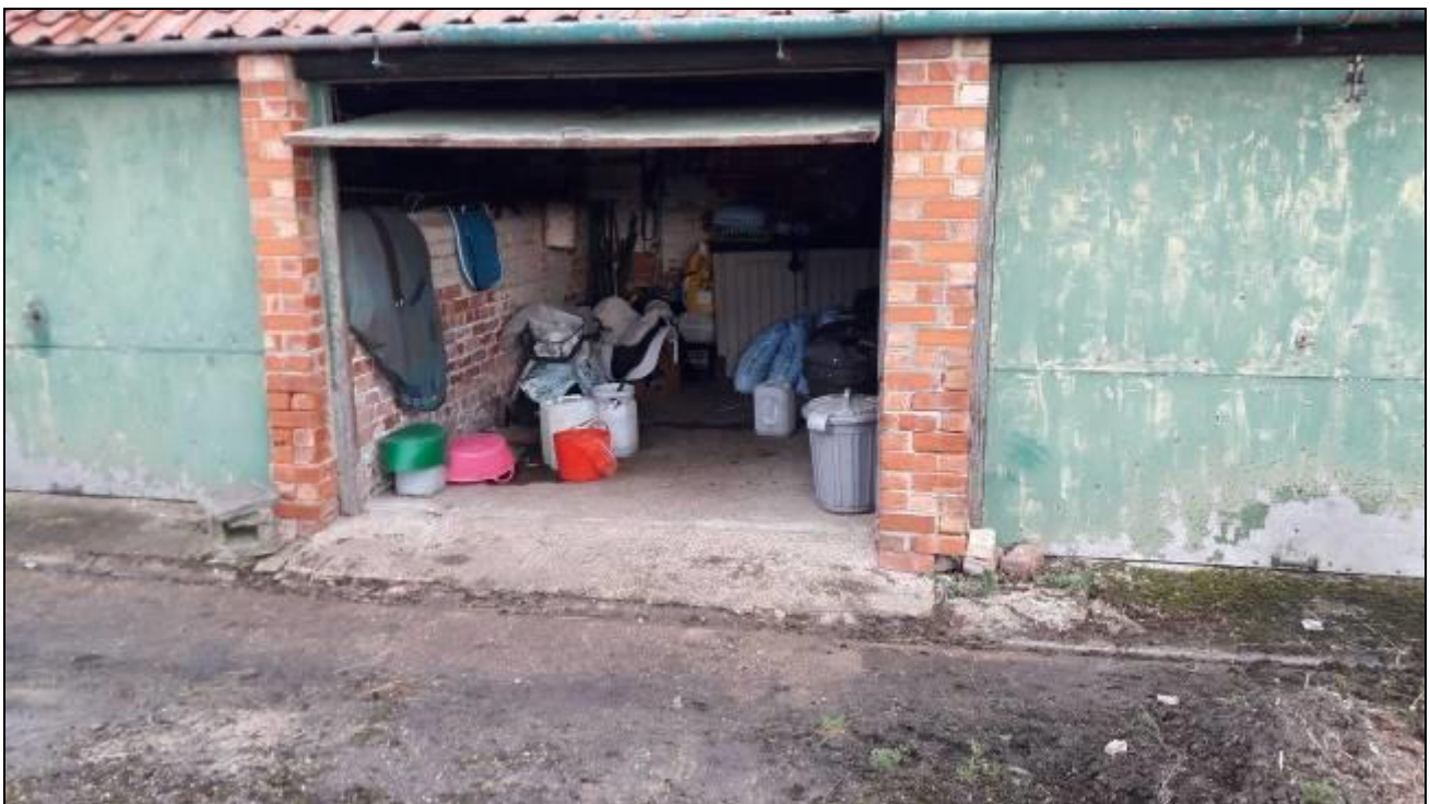
Fig 13 - view to the north of the lock-up garages, with concrete floors
