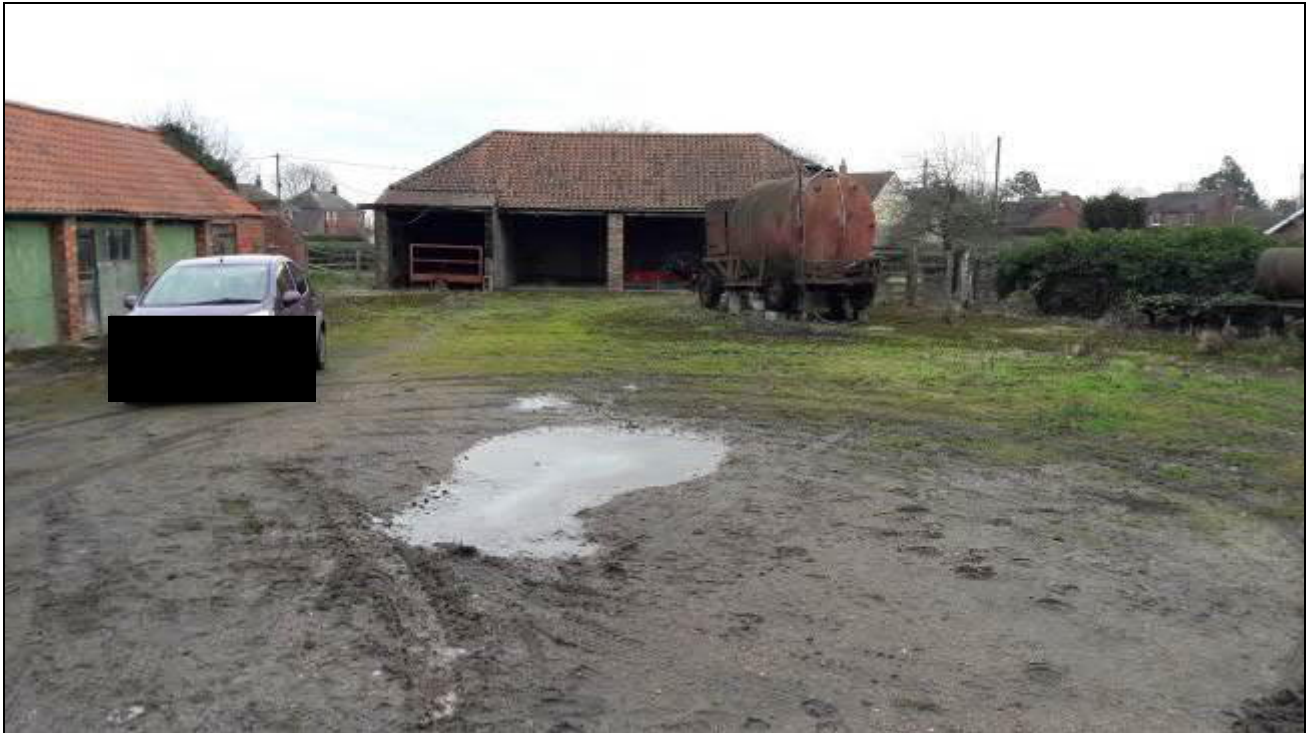
Fig 12 - view to the east of the sheds on the east side
