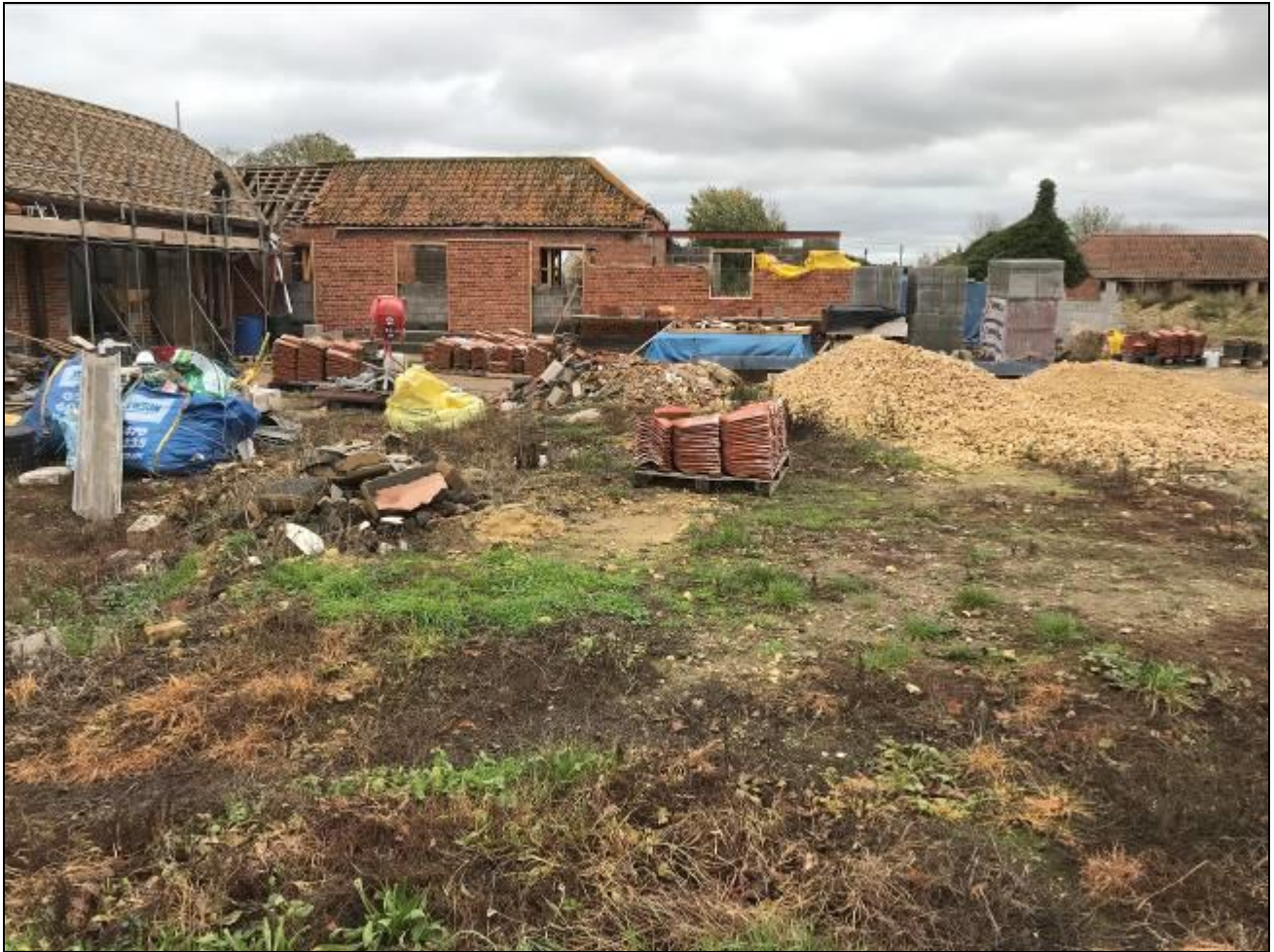
Fig 8 – position of dutch barn after removal
